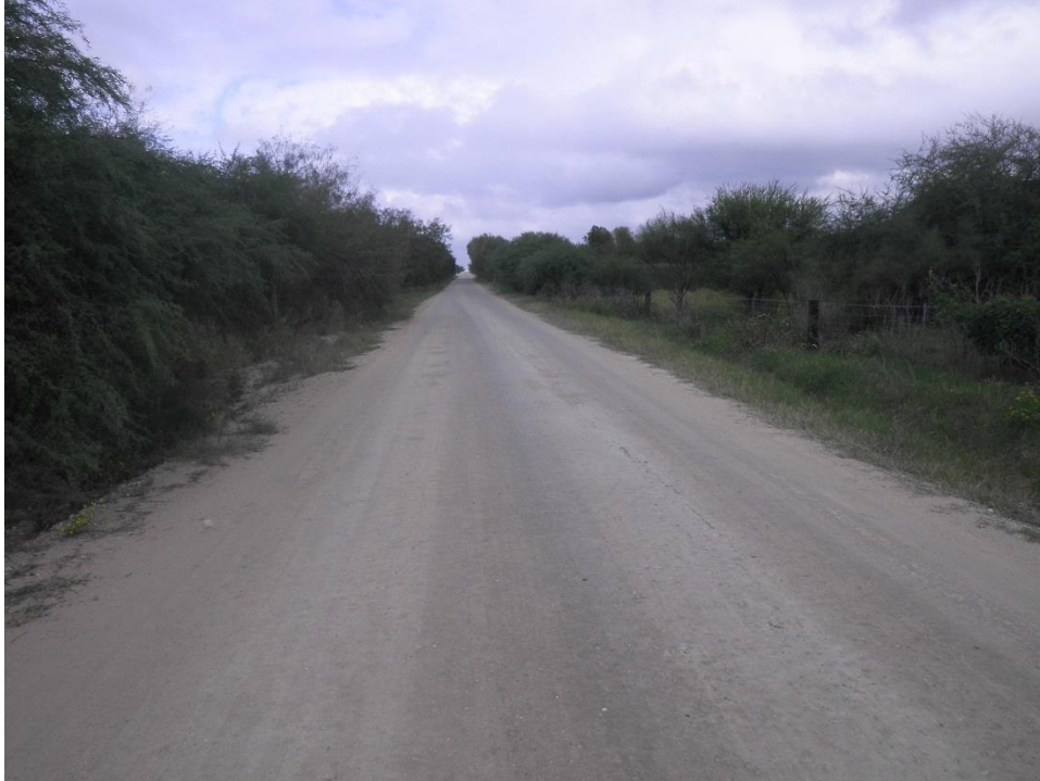
Figure 2. View north along CR 10 from south end of APE.
