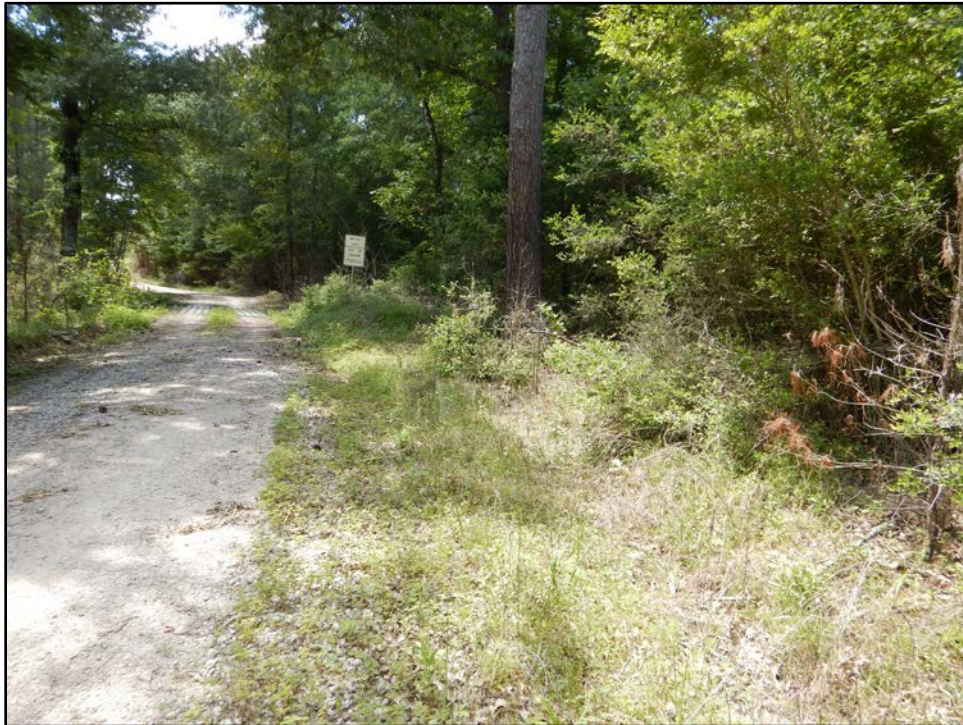
Figure 2. Photo of existing bridge (at the sign) and ROW facing east.
