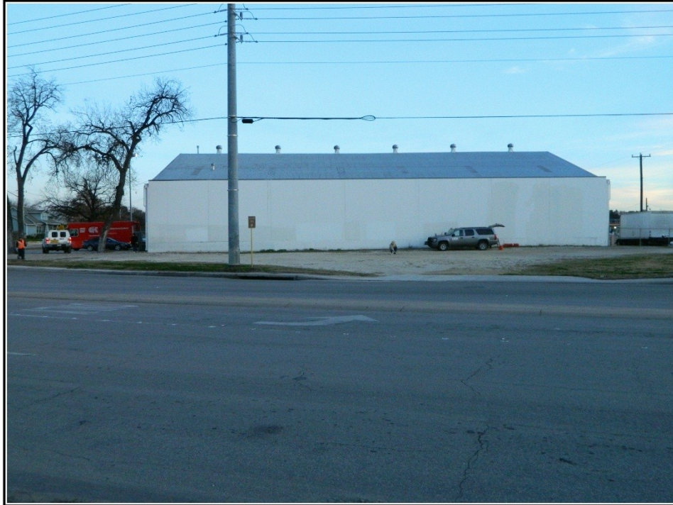
Figure 1-2. General view of the APE facing north.
