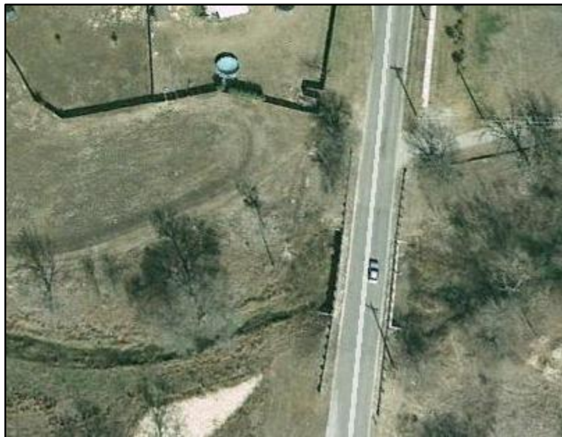
Figure 1-6. View of northwest side of Plum Creek in 2009. Note fill that forms the levy berm.
