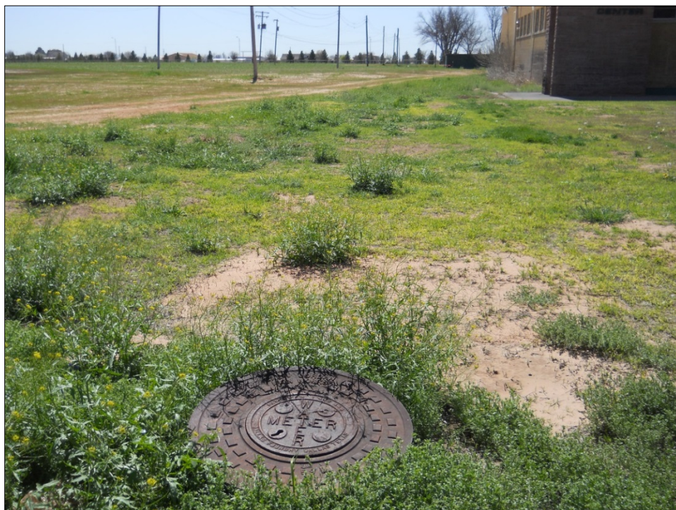
Figure 4-5. Photograph Showing Recent Sewer Line Disturbance.
