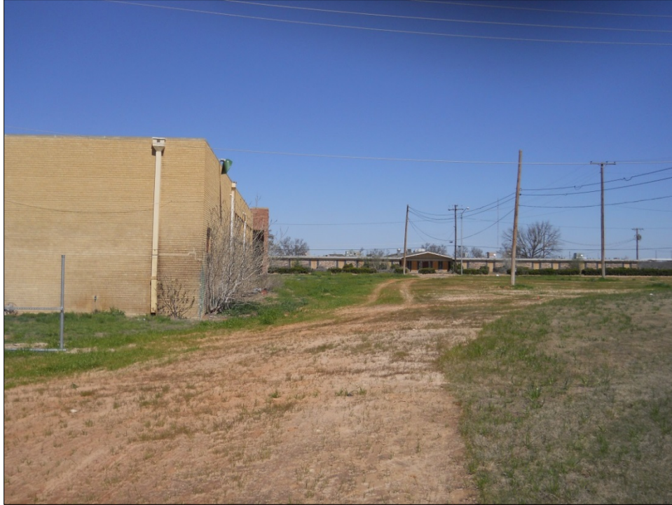
Figure 4-2. Overview of APE from Southeastern Corner, Facing Northwest.
