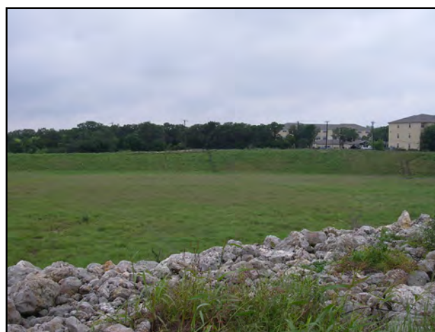
Figure 5.5. Proposed Wurzbach Parkway right-of-way west of Vista del Norte near site 41BX184 facing west and illustrating major land modifications associated with the flood control dam construction. Rock pile in the foreground is the same one seen in the background of Figure 5.4.
