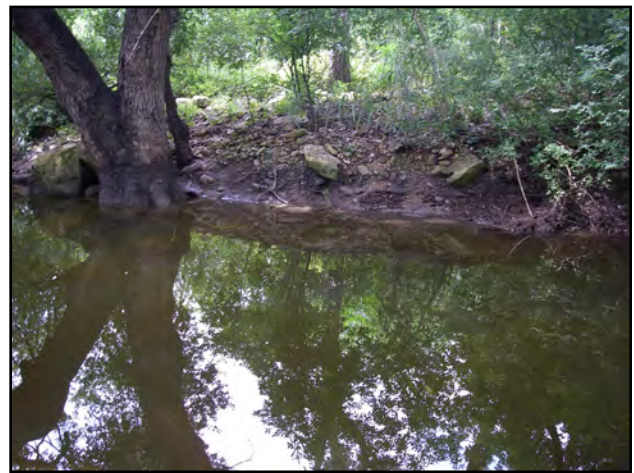
Figure 5.11. Cutbank along Salado Creek on the west side of U.S. 281, facing south.
