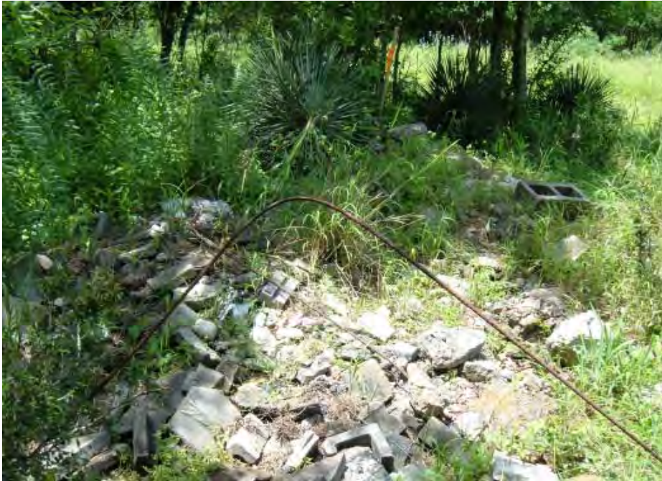
Figure 1. Construction debris and disturbed surfaces west of CSN 228+44.
