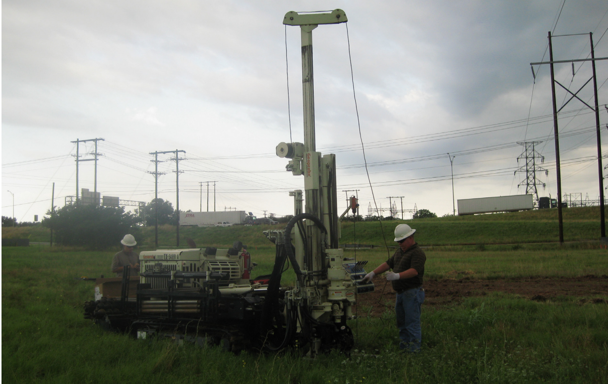
Figure 7. South-southwest view of coring by the Geoprobe near Trench 4.
