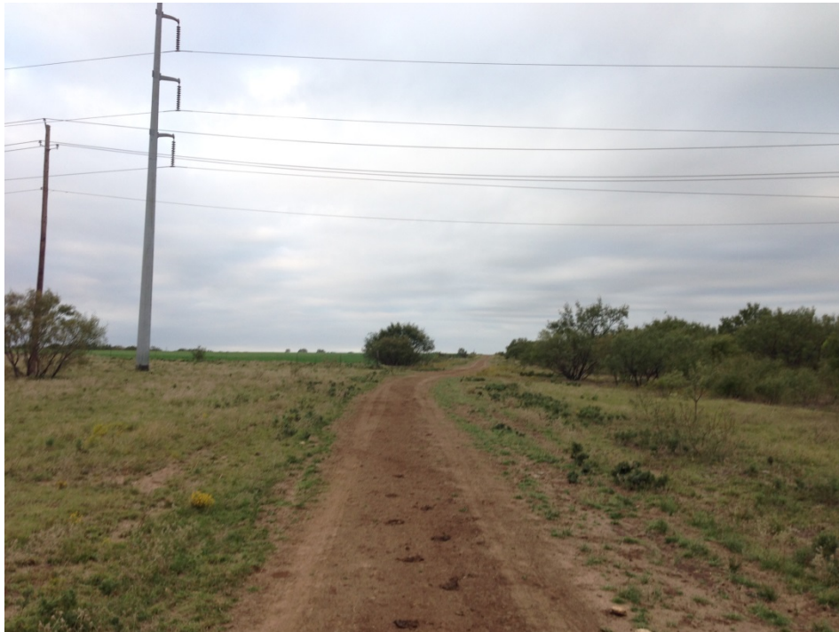
FIGURE 3 EXISTING TRANSMISSION LINE, DISTRIBUTION LINE, AND DIRT ROAD IN PROJECT AREA, FACING WEST.
