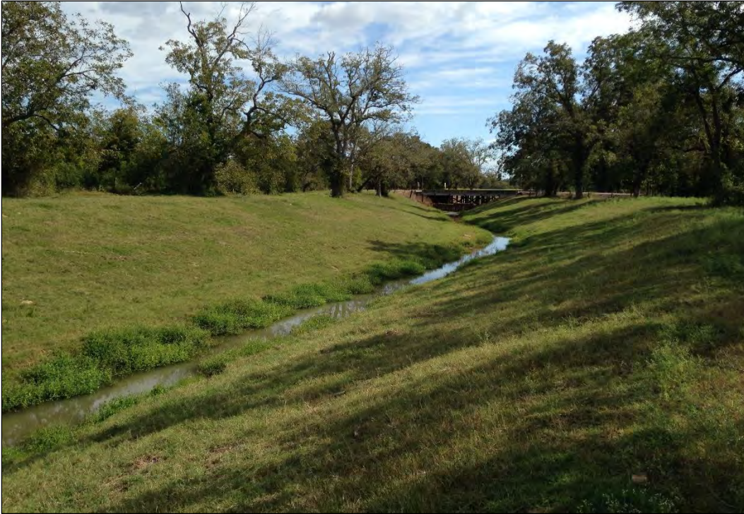
Figure 12. Typical View of Brookshire Creek Channel (Facing South)
