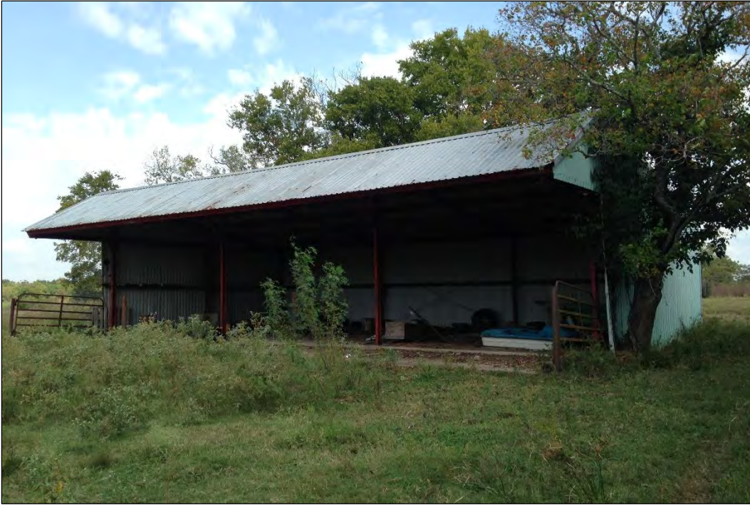
Figure 39. Front (Western) Façade of Metal Barn/Equipment Shed (Facing Northeast)
