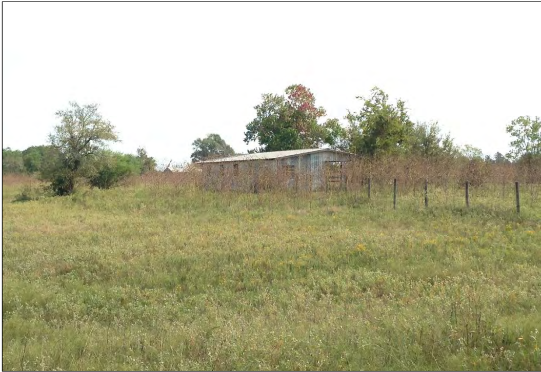
Figure 41. View of Wood-Paneled Barn/Equipment Shed (Facing Southeast)
