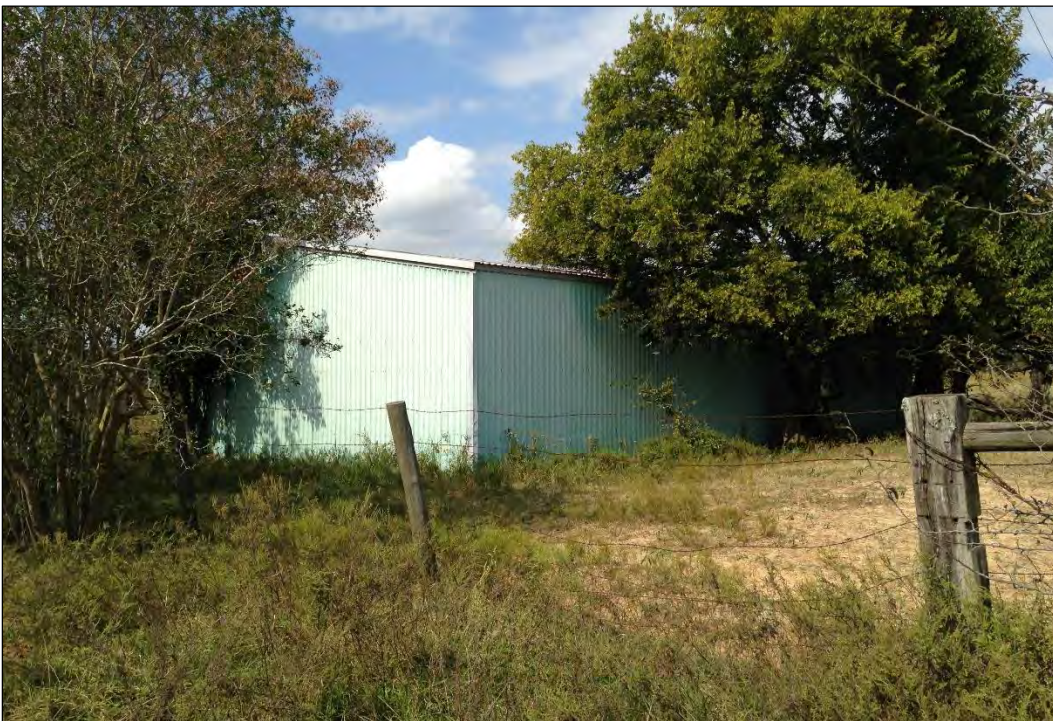
Figure 40. Back (Eastern) and Side (Southern) Façades of Metal Barn/Equipment Shed (Facing Northwest)
