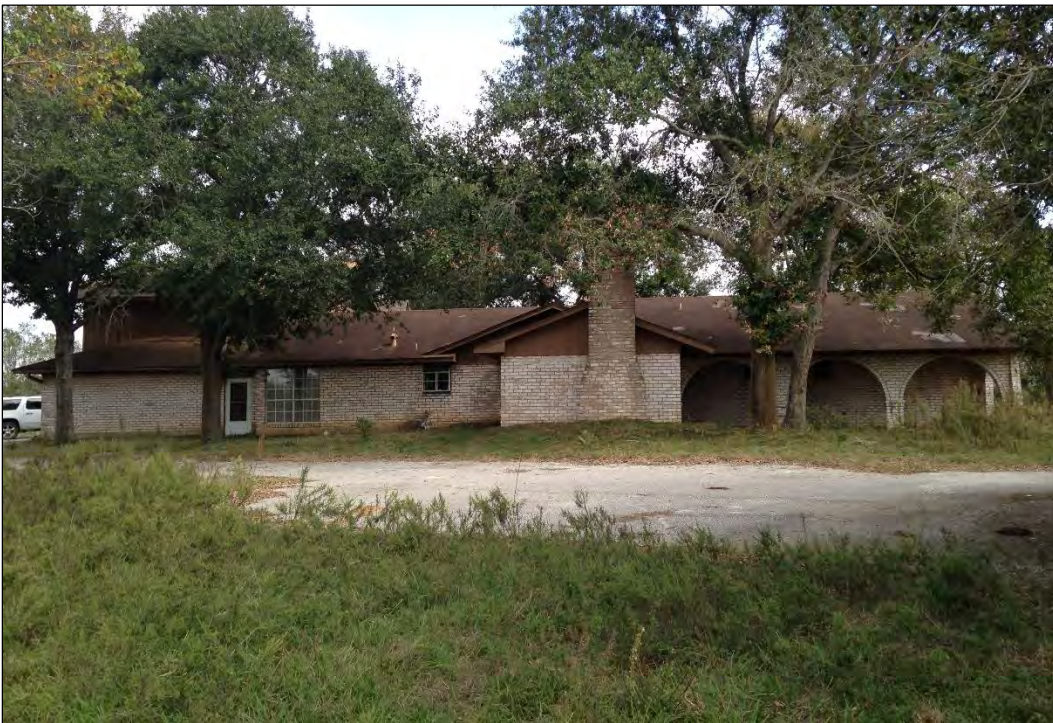
Figure 36. Back (Western) Façade of Residence (Facing East)
