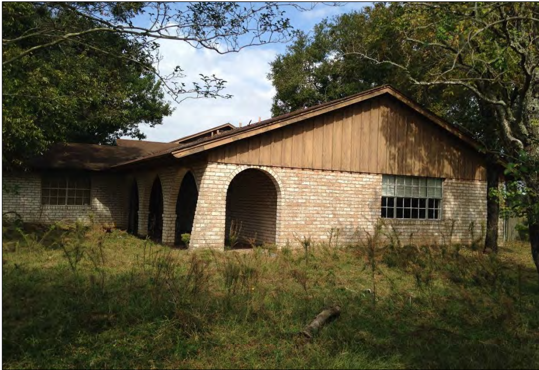
Figure 37. Side (Southern) Façade of Residence (Facing Northeast)
