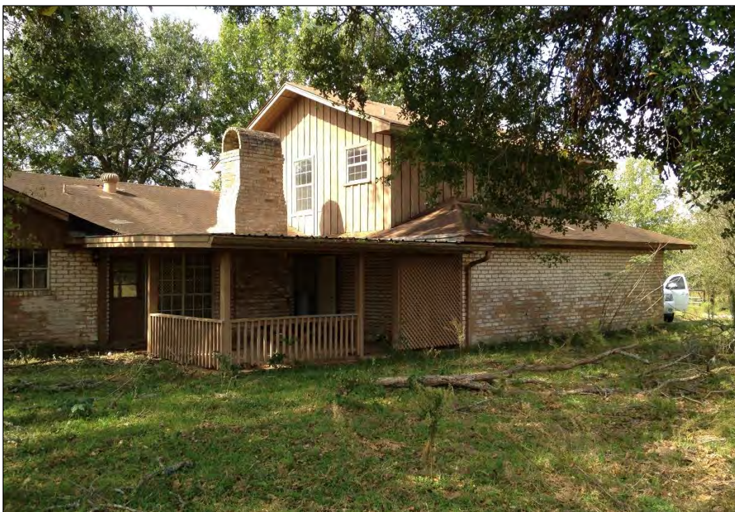
Figure 38. Front (Eastern) Façade of Residence (Facing Northwest)
