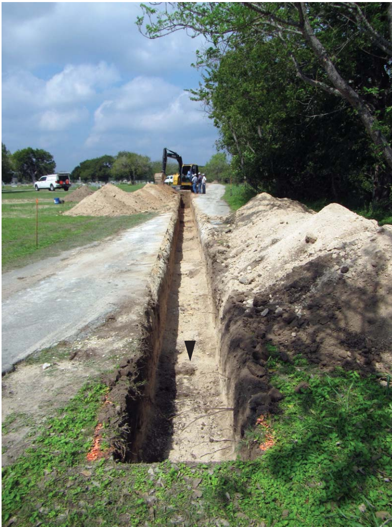
Figure 13. View of Trench 5 looking northwest down the project corridor. The southeast end of the trench is in the foreground, and the trackhoe is near the northwest end. The arrow points to Borehole 5, a clay-filled circle in the bottom of the trench.
