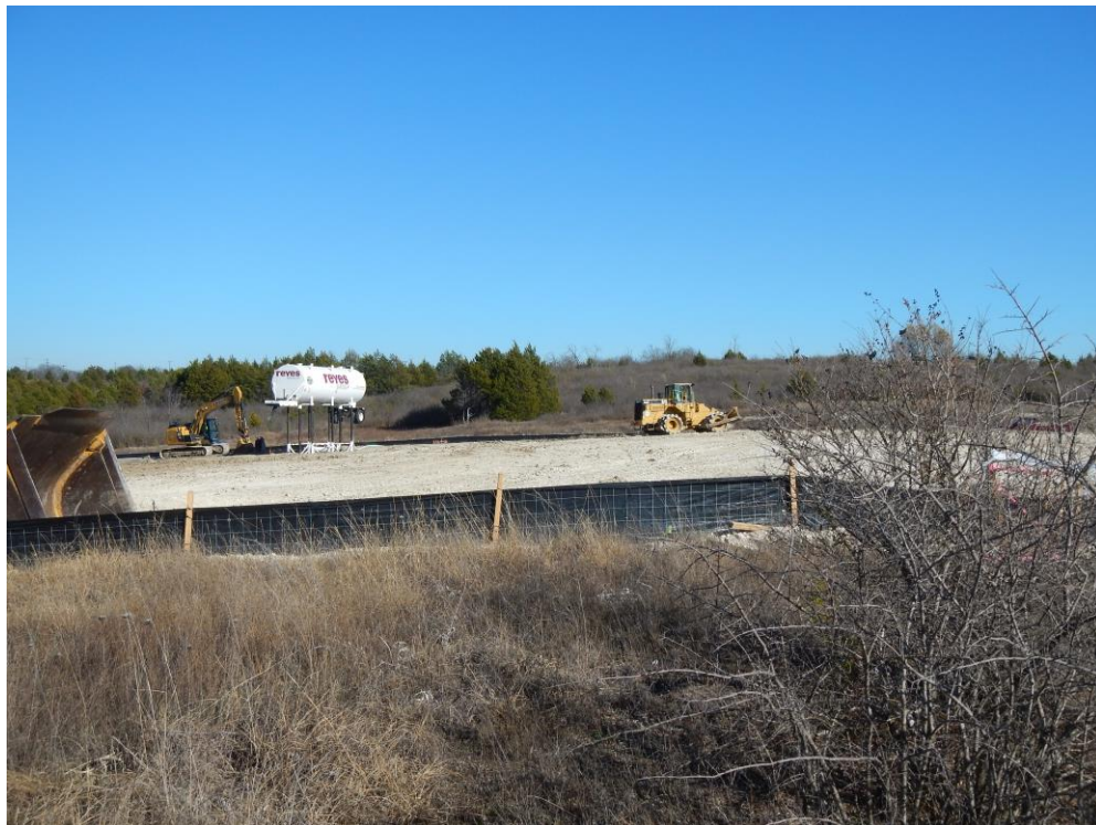
Figure 4. DART construction occurring on abutting property to the east; facing east
