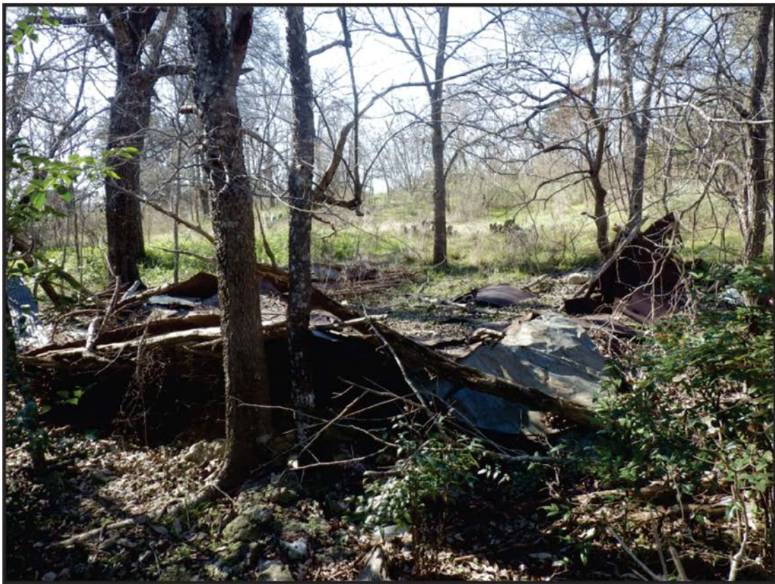
Figure 11. Feature 1, collapsed structure, looking north.
