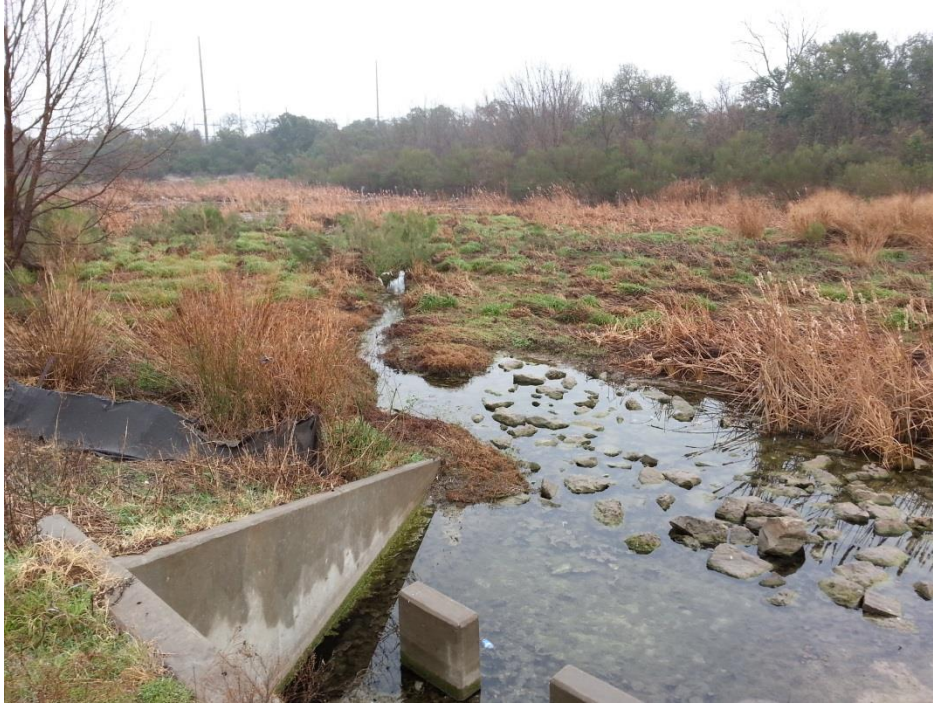
Figure 4. View northeast at Lake Creek floodplain adjacent to APE near mapped location of 41WM971. Taken from on top of 2-m-high artificial embankment. Note drainage structure (outlet from detention pond).
