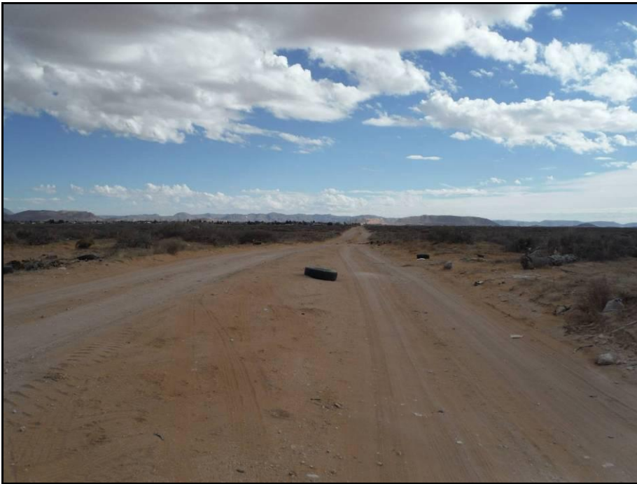
Figure 6. Paved Greg Dr. and unpaved road going west.
