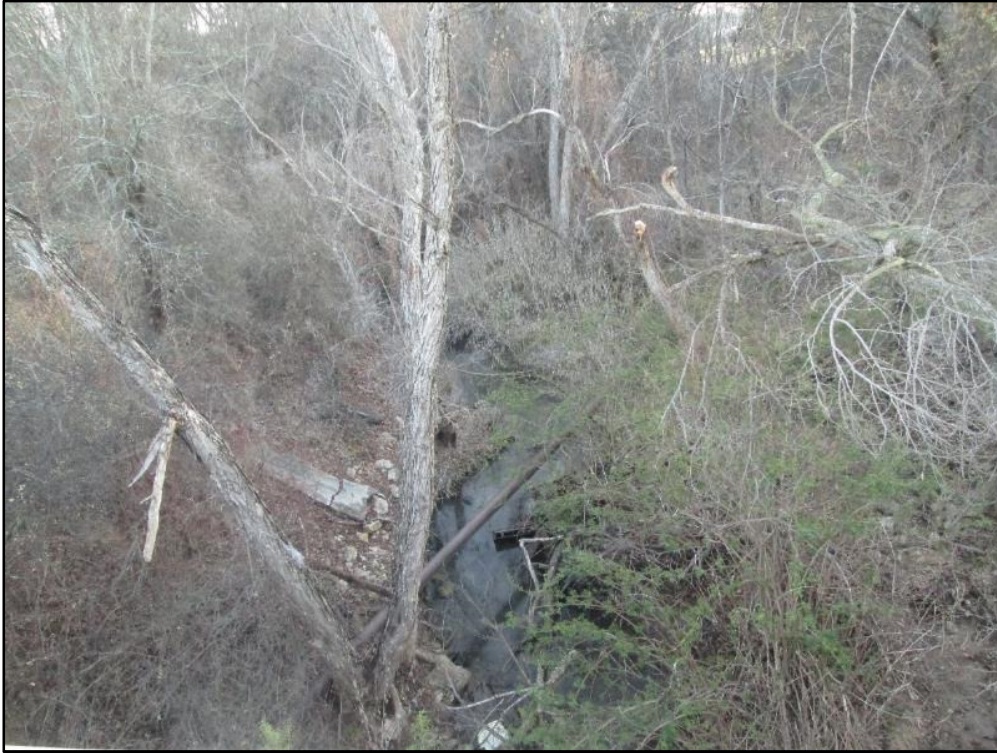
Figure 4. Overview of upstream at Hog Creek at FM 8, facing north. Note buried pipelines.
