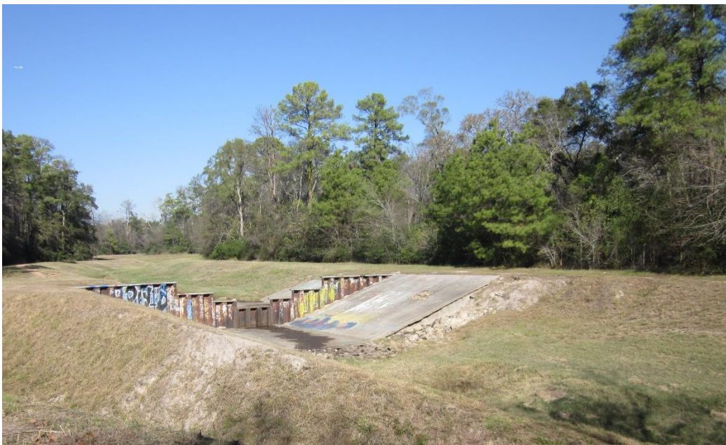
Figure 5-3. View of flood control measures along Schultz Gully, looking northeast.
