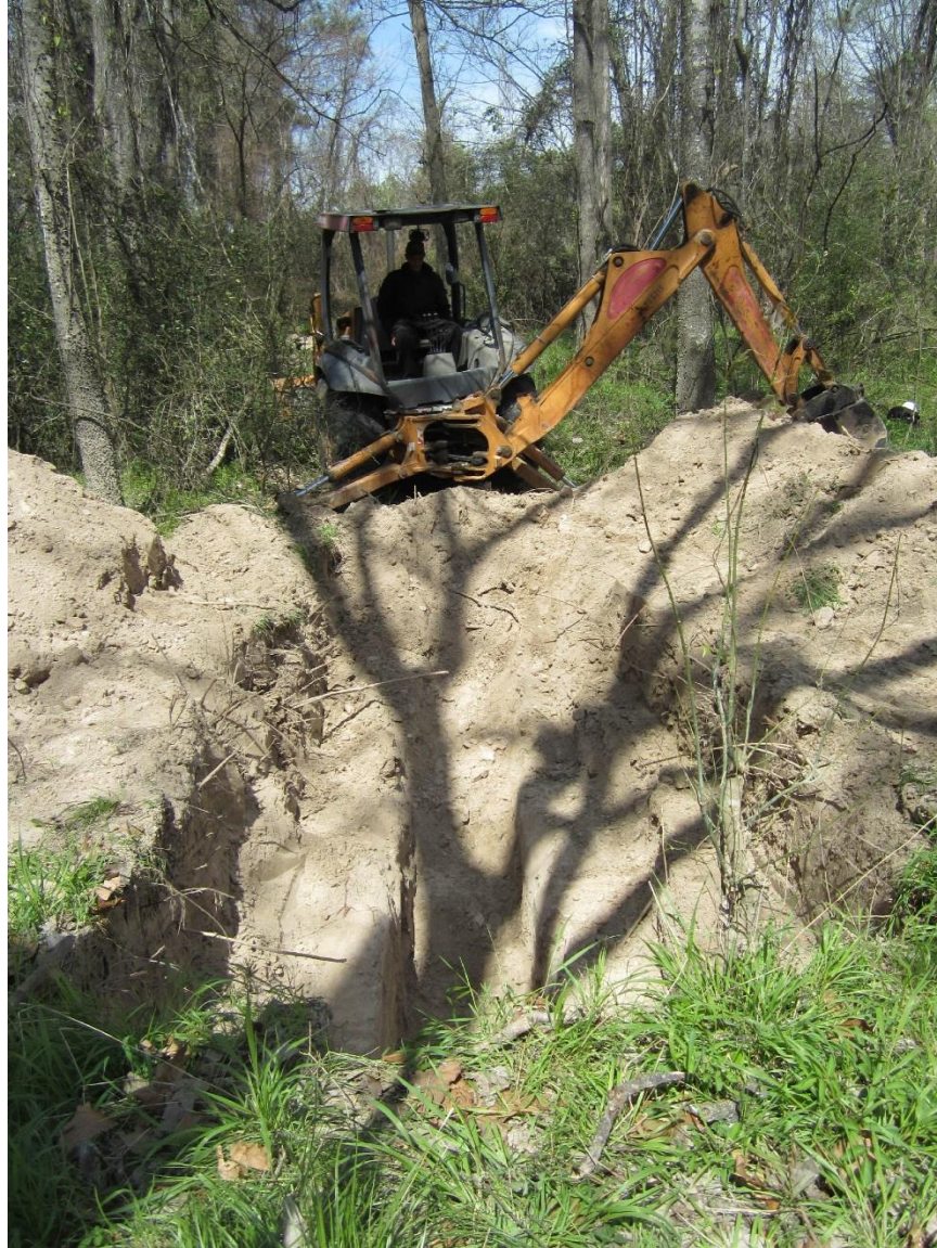
Figure 5-15. View of Trench 2 Excavation in progress, looking north.
