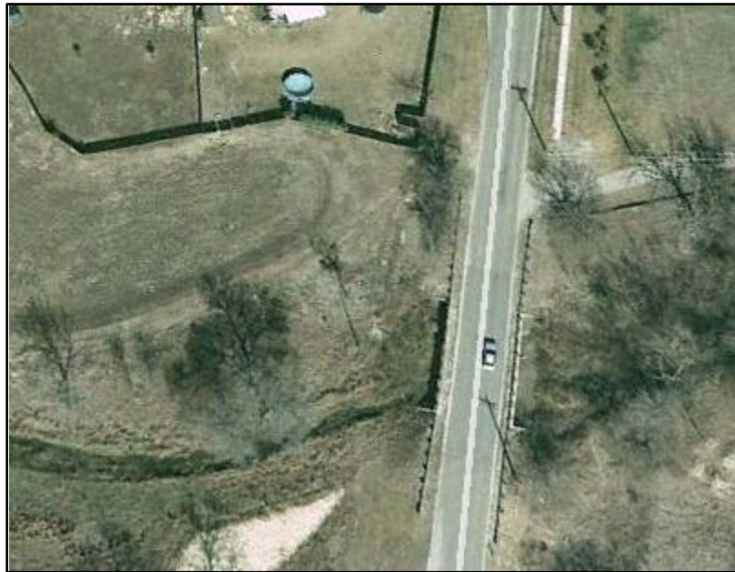
Figure 1-6. View of northwest side of Plum Creek in 2009. Note fill that forms the levy berm.
