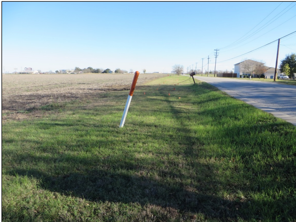
Figure 1-3. West side of the ROW facing northeast. Note utility pole and flags which indicate buried telecommunications lines.
