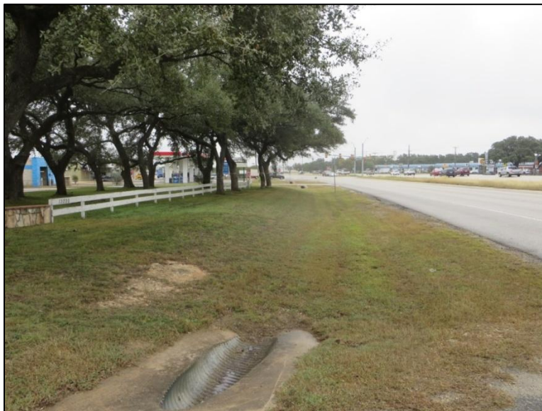
Figure 2-1. Typical setting along ROW. Note exposed bedrock and concrete culvert.
