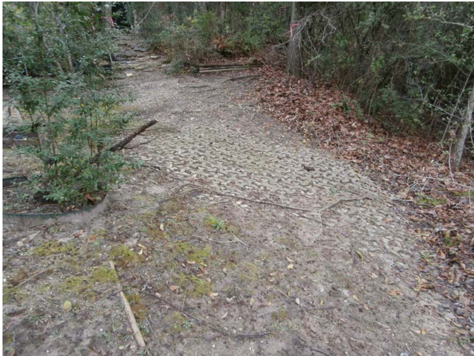
Figure 6. "Tri-lock" bank stabilizer.
