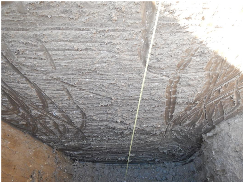
Figure 5. Bottom of south wall profile in Trench 1. Note water seepage at bottom.
