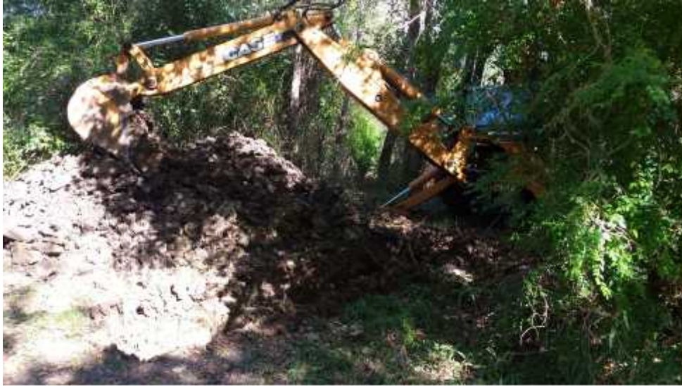
Photo #3: Northerly view of ongoing BHT 1 excavation.
