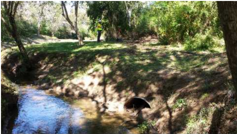
Photo #4: Northwesterly view of Armand Bayou picturing an approximately two-foot diameter culvert emerging from the left bank. BHT 1 was located approximately 25 m to the right (north) of the bayou.
