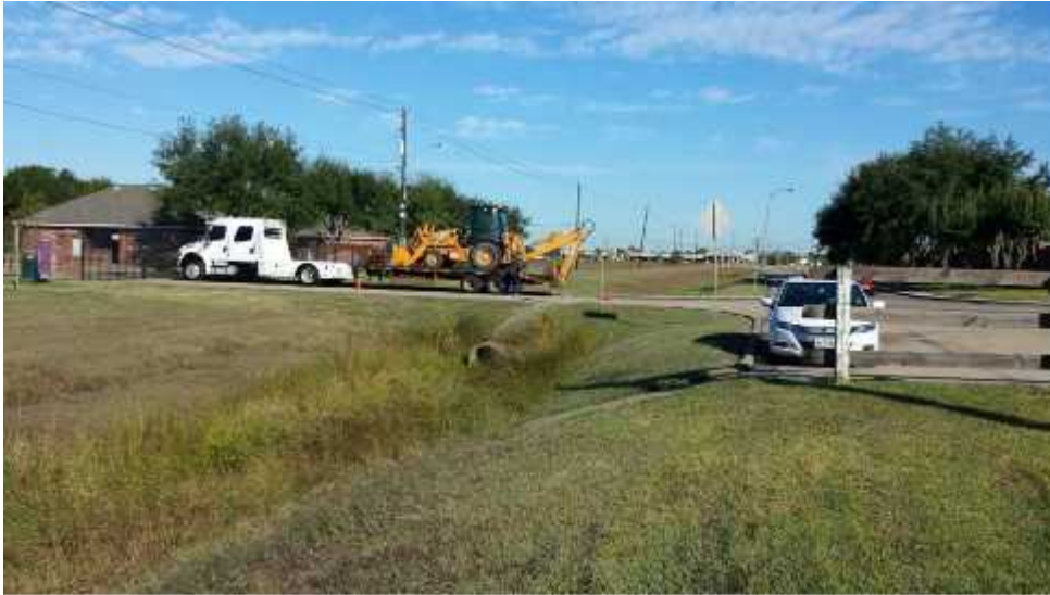
Photo #1: The current (as of November 18, 2012) terminus of Center Street, and the channelized drainage on the west along the west side of the area of potential effect (APE) north of Armand Bayou.
