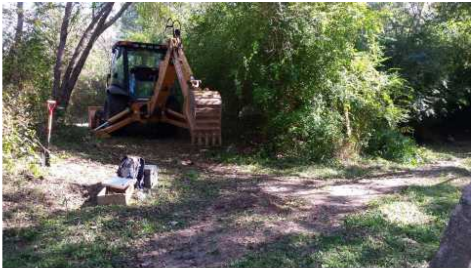
Photo #2: Northerly view of the beginning of Backhoe Trench (BHT) 1 excavation.
