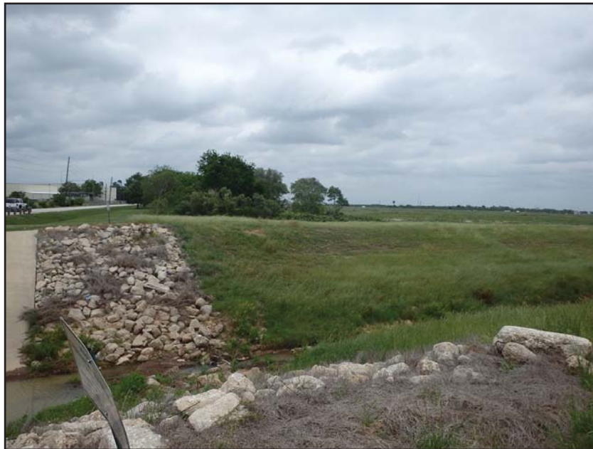
Plate 2. Overview of Project Outfall 1 showing disturbance. View is to the northeast.
