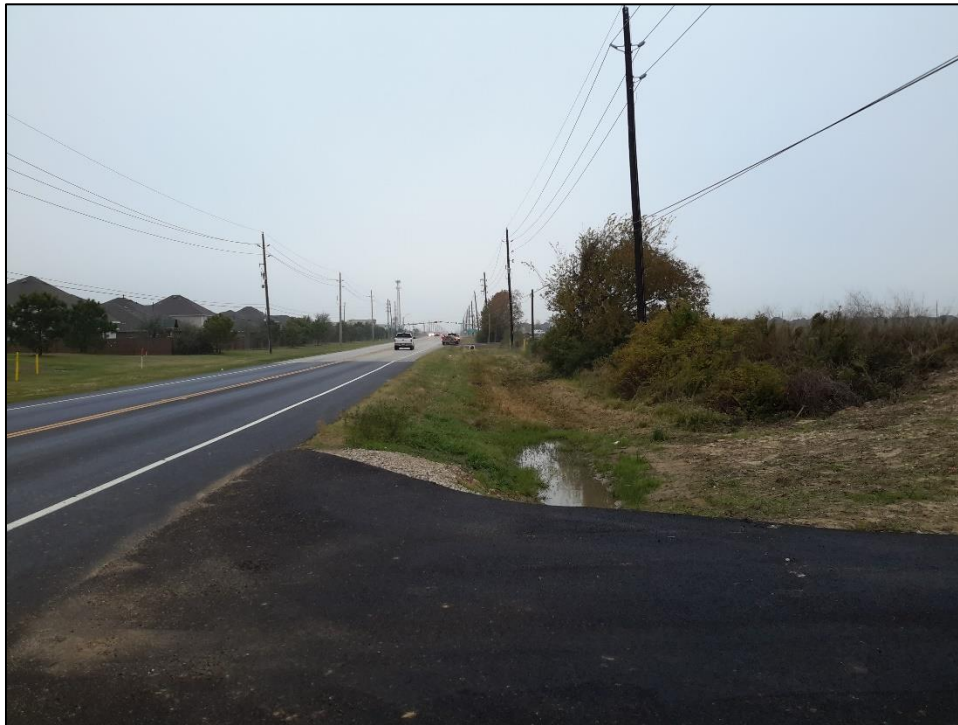
Figure 5. Overview of typical roadside impacts and marked utilities alongside FM 1463, facing south.
