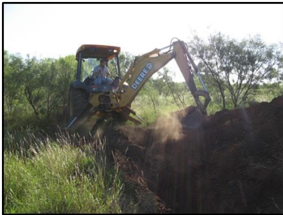
Exhibit 3. Excavation of Backhoe Trench by the City of Ballinger
