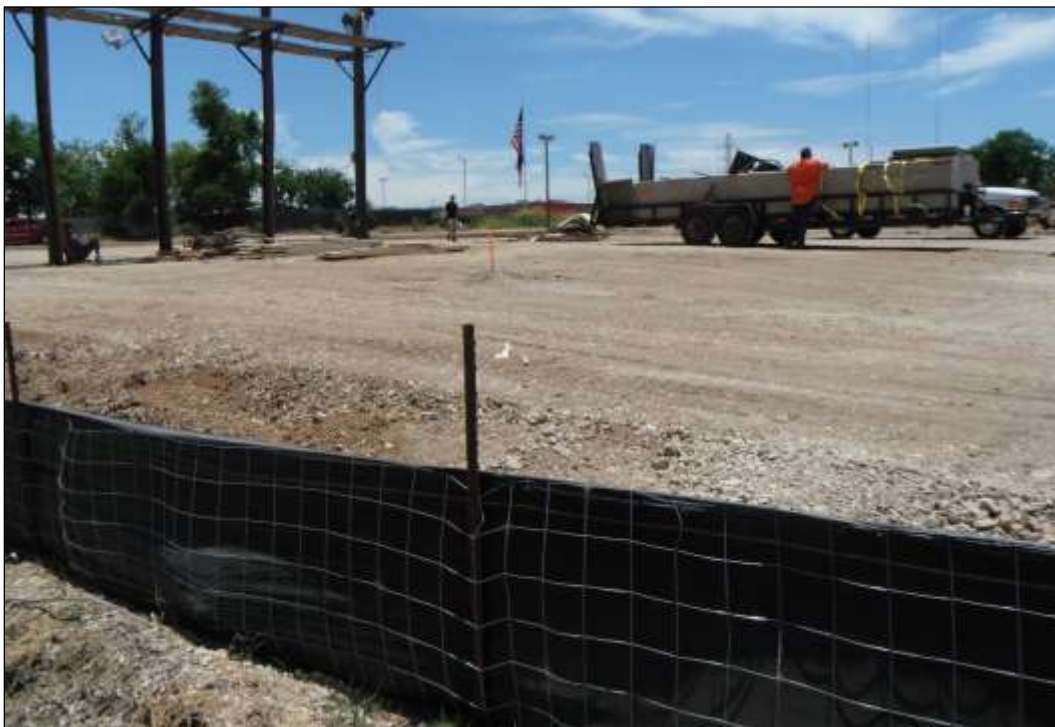
Figure 9. Contractor Yard at Holbrook Road and Austin Highway (Facing Southeast)
