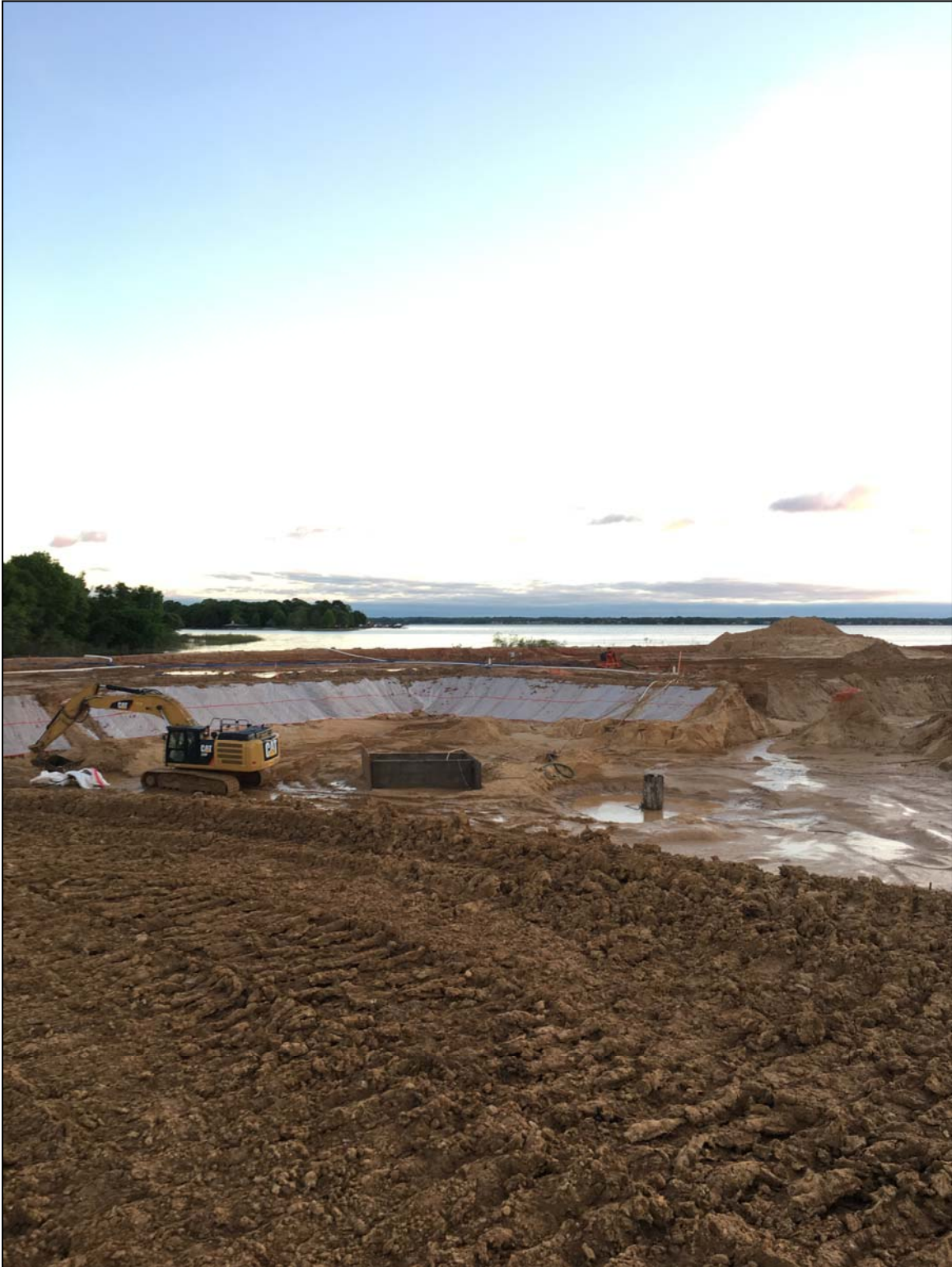
Figure 3. View of the pump station site in April 2017, facing northeast.
