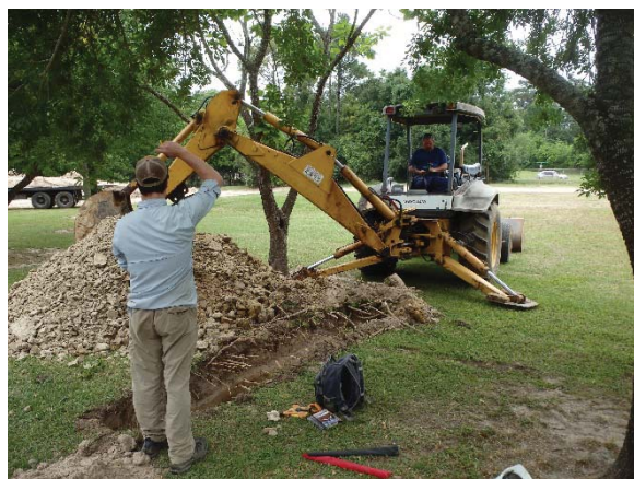
Figure 5-2. Overview of north APE. View is to the northwest.
