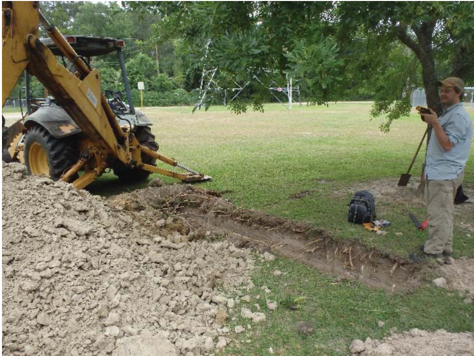
Figure 2-2. North bore pit location. View is to the northeast.
