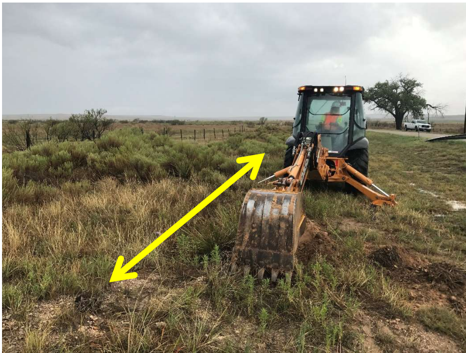
Figure 6. Overview of BHT 5 showing setting on western side of APE with artificial berm along ROW margin (denoted by bi-pointed arrow), downcut drainage ditch that has likely removed much of the archeological potential, and fill section that raises existing roadway above surrounding landscape.
