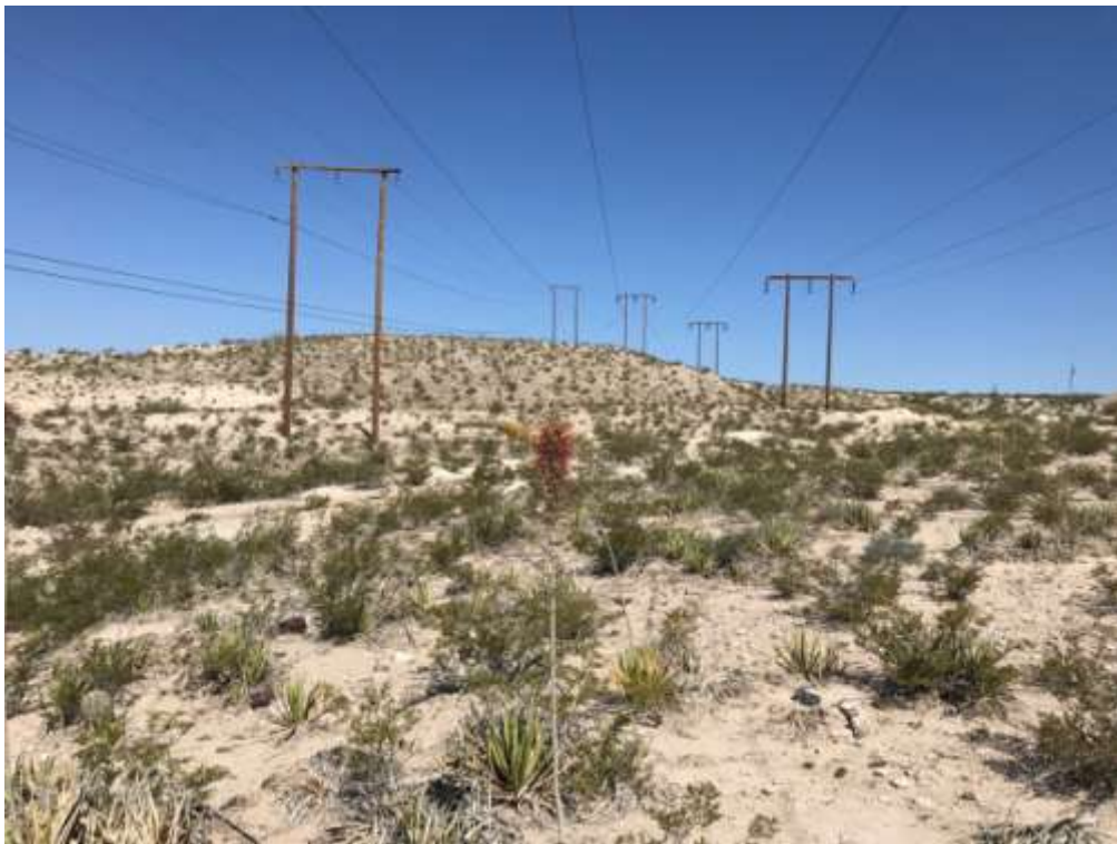
Figure 11. Bladed areas noted throughout northern portion of project area (facing southeast).
