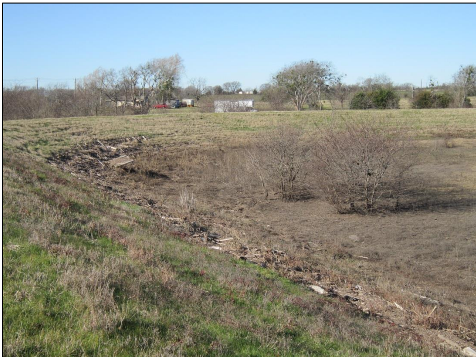
Figure 9. West end of earthen dam, within exposed inundation area. Facing west.
