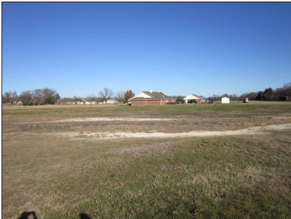
Figure 19. View across northern part of auxiliary spillway, showing excavated zone and exposed bedrock. Facing north.
