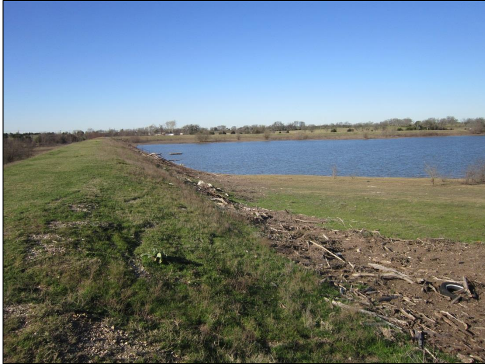
Figure 6. Overview of earthen dam. Facing southwest.
