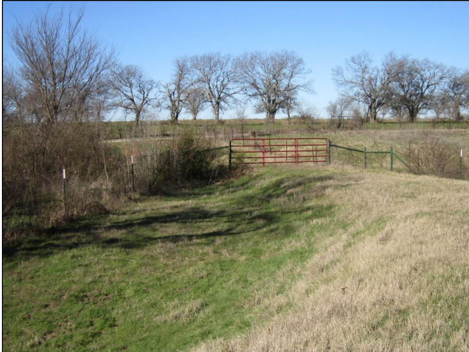
Figure 11. Entrance point at northwest corner of earthen dam structure. Facing west.
