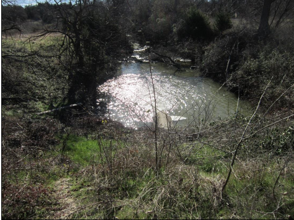
Figure 8. View of outlet pipe and plunge basin below dam. Facing southeast.
