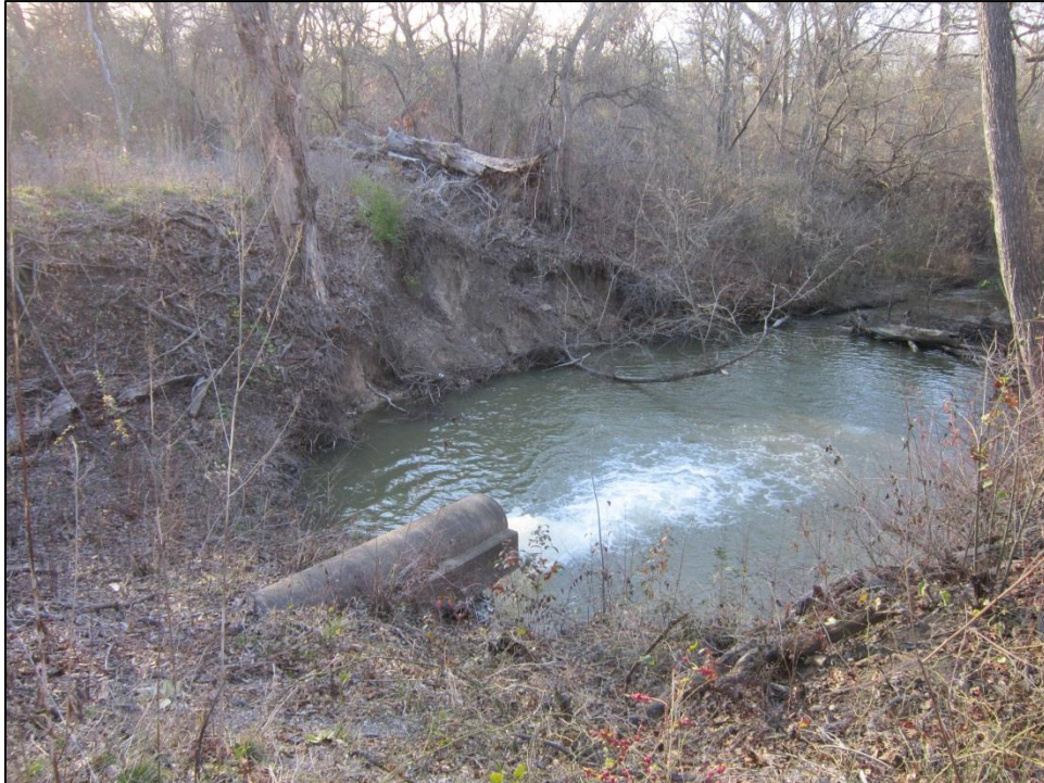
Figure 17. View of outlet pipe and plunge basin below dam. Facing south.
