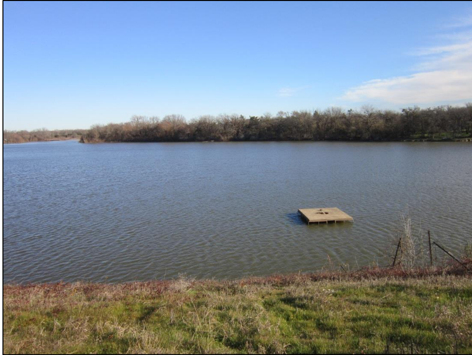
Figure 18. Dam inlet inside the inundation area. Facing north.
