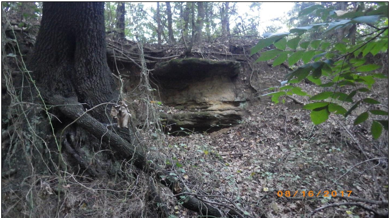
Figure 13. West bank of Bakers Branch showing large outcrop of sandstone. The top of the picture is the elevation of the running trail.
