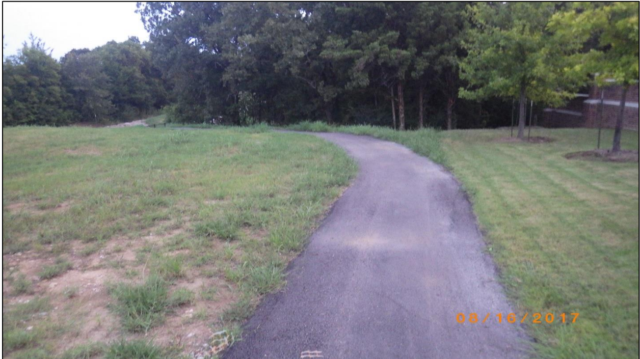
Figure 6. Asphalt trail connecting new eastern subdivision to the concrete running trail. View is to the north.
