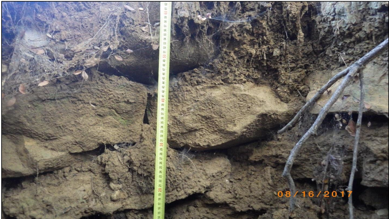
Figure 17. Interior of cistern/well (41DN604) wall showing the sandstone blocks.
