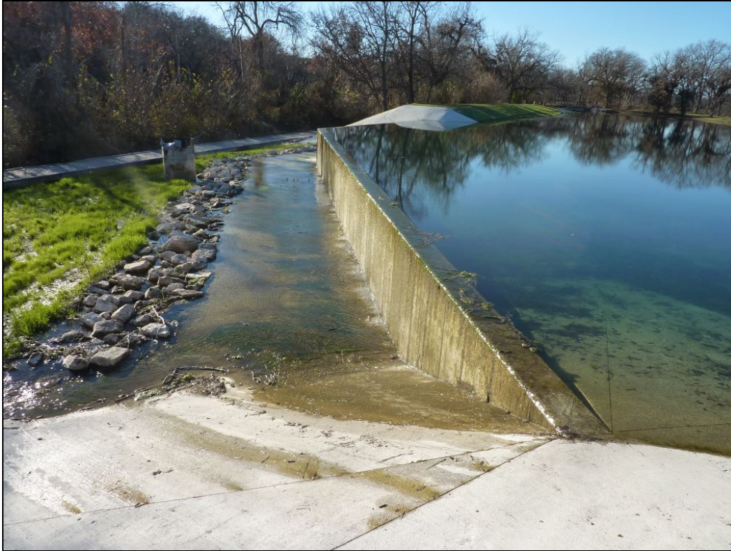
Figure 9. View of the concrete dam built over the Gan's Dam.
