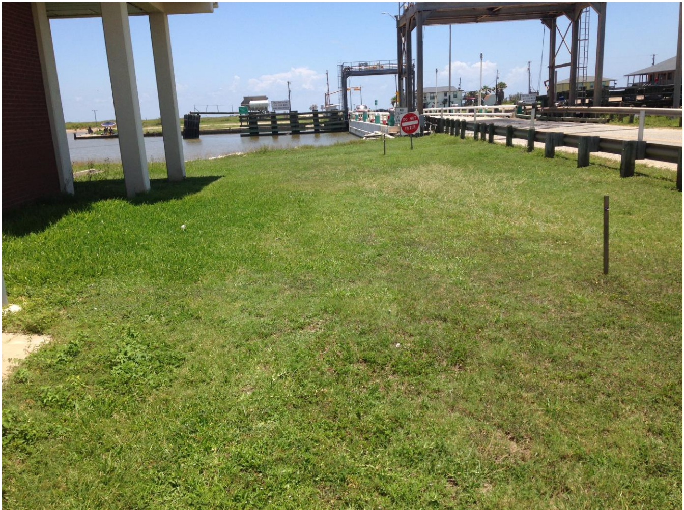
Figure 5. Well-maintained ROW within the APE in NE Quadrant; opposite side of GIWW is a cleared vacant lot in the SE Quadrant. This is the side where circular bridge ramps will be located
