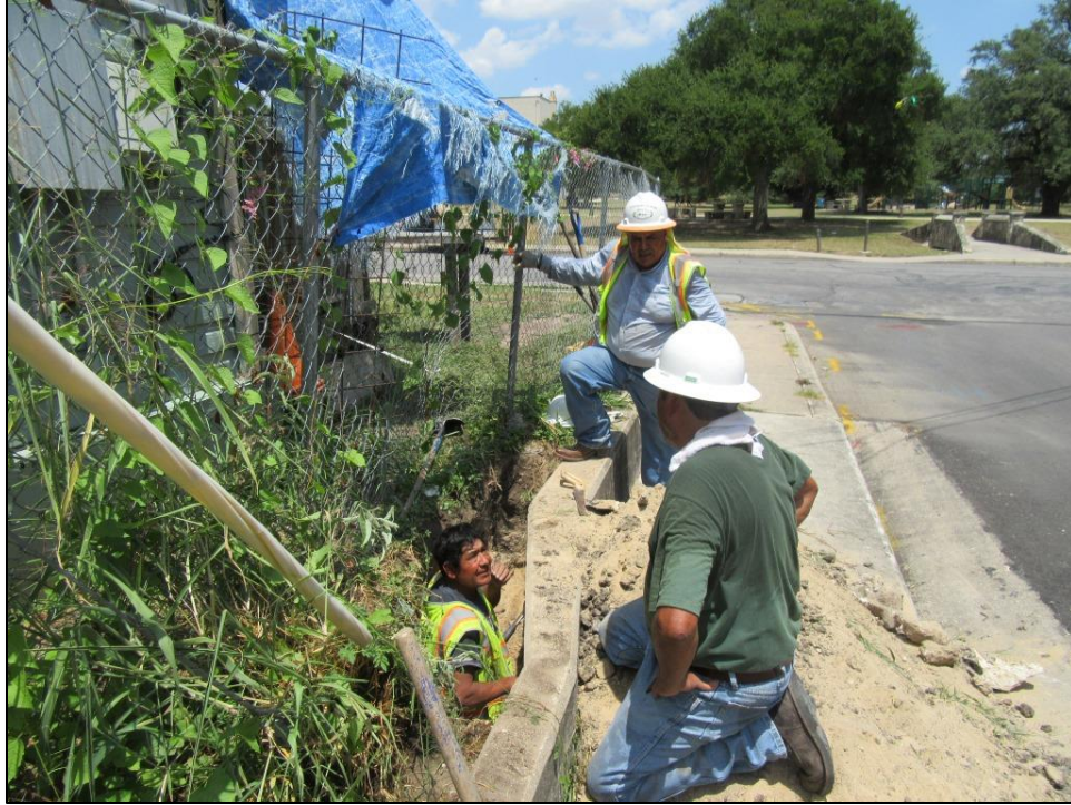
Figure 7. Excavation of trench along Kempkau.
