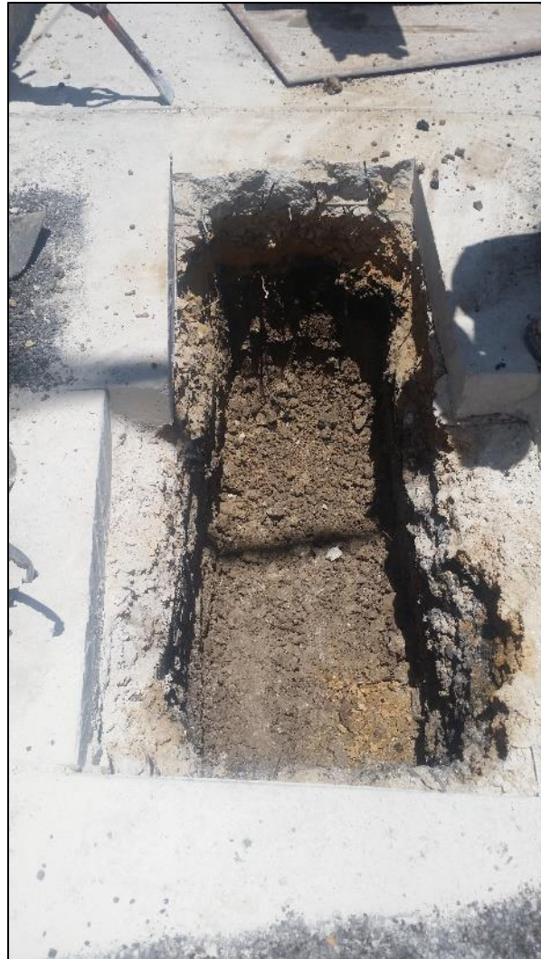
Figure 6. Overview of BP 8, typical of what was seen in BPs 6–10.
