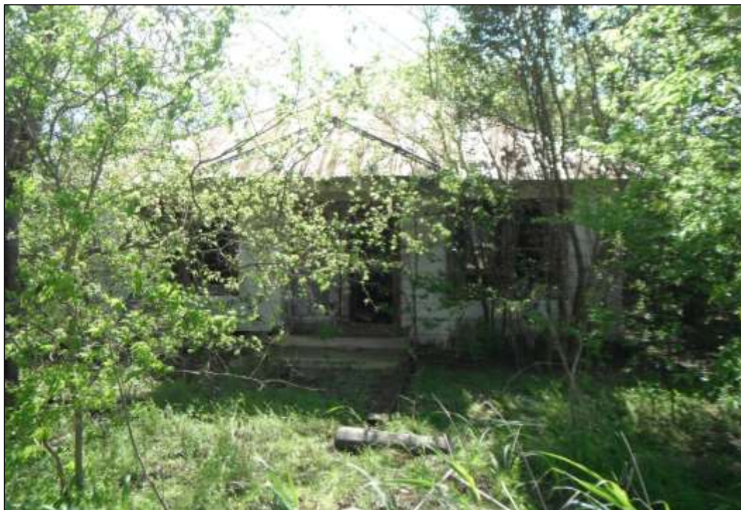
Figure 6-3. Structure W1-A (41HY536)—Front of House (Facing Southeast)
