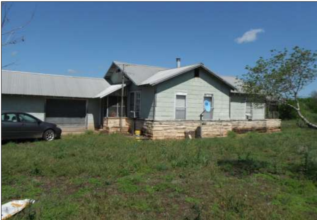
Figure 6-38. Structure W4-A (41HY539)—Southeastern Side of House (Facing North)
