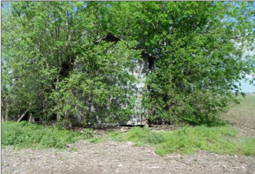
Figure 6-7. Structure W1-B (41HY536)—Side of Barn (Facing Southwest)
