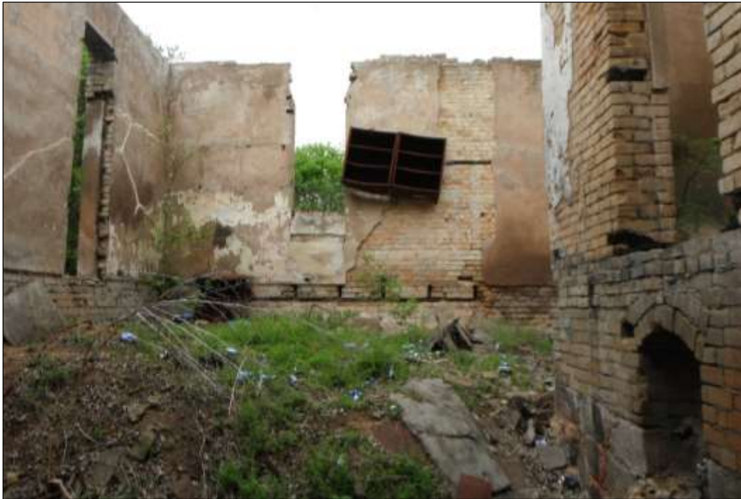
Figure 6-63. Structure W6-A (41HY541)—Northwestern Room Interior from Basement (Facing Northwest)
