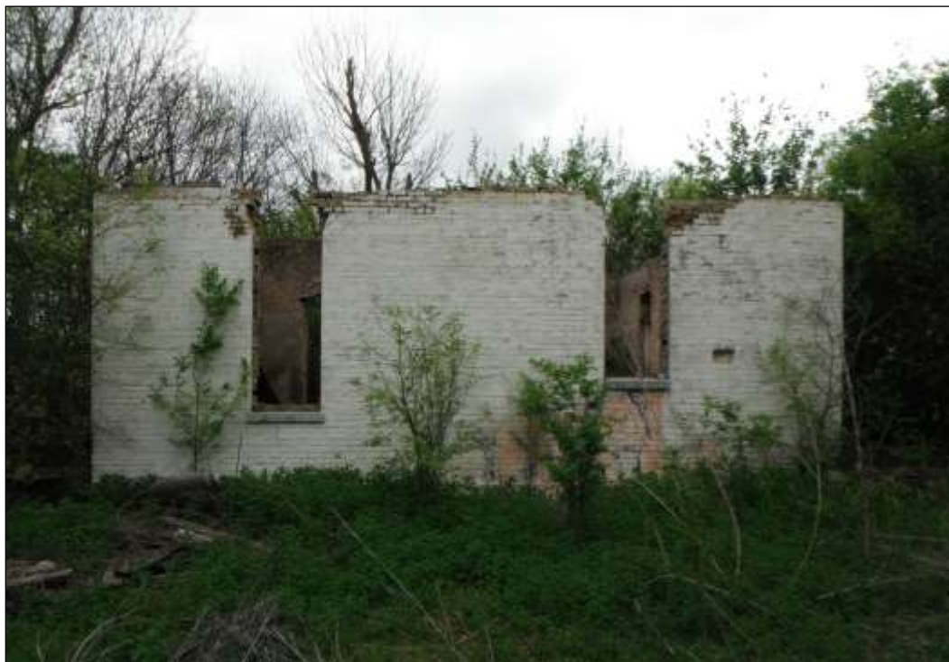
Figure 6-57. Structure W6-A (41HY541)—Northwestern Side of House (Facing Southeast)
