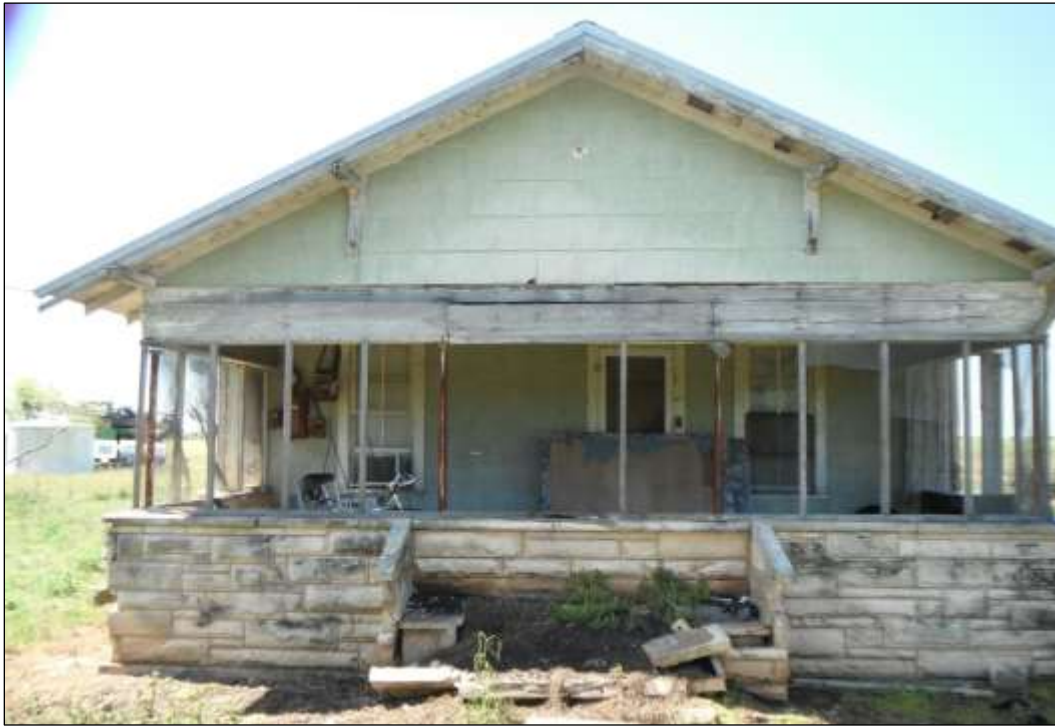
Figure 6-36. Structure W4-A (41HY539)—Front of House (Facing Southwest)
