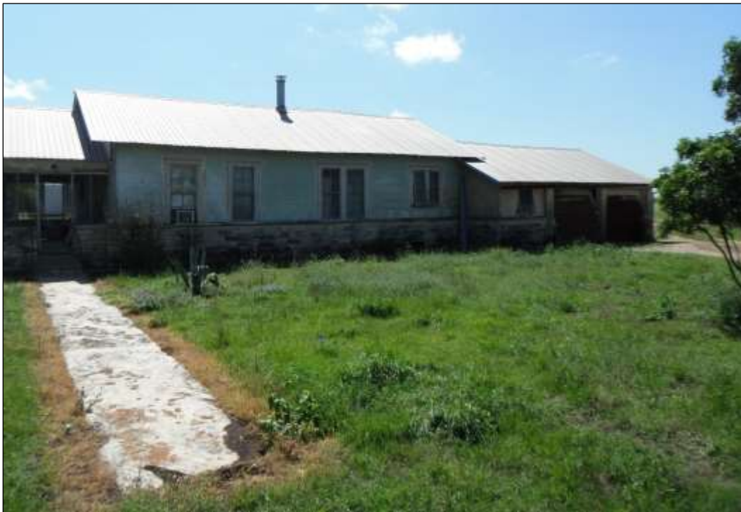
Figure 6-37. Structure W4-A (41HY539)—Northwestern Side of House (Facing Southeast)
