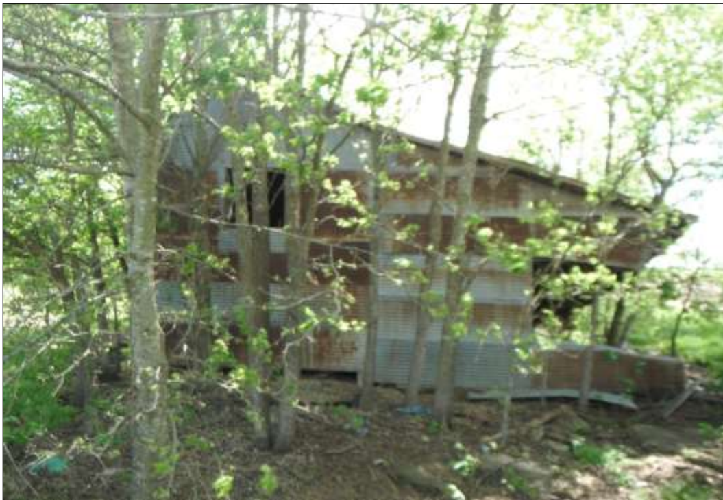
Figure 6-6. Structure W1-B (41HY536)—Side of Barn (Facing Northeast)
