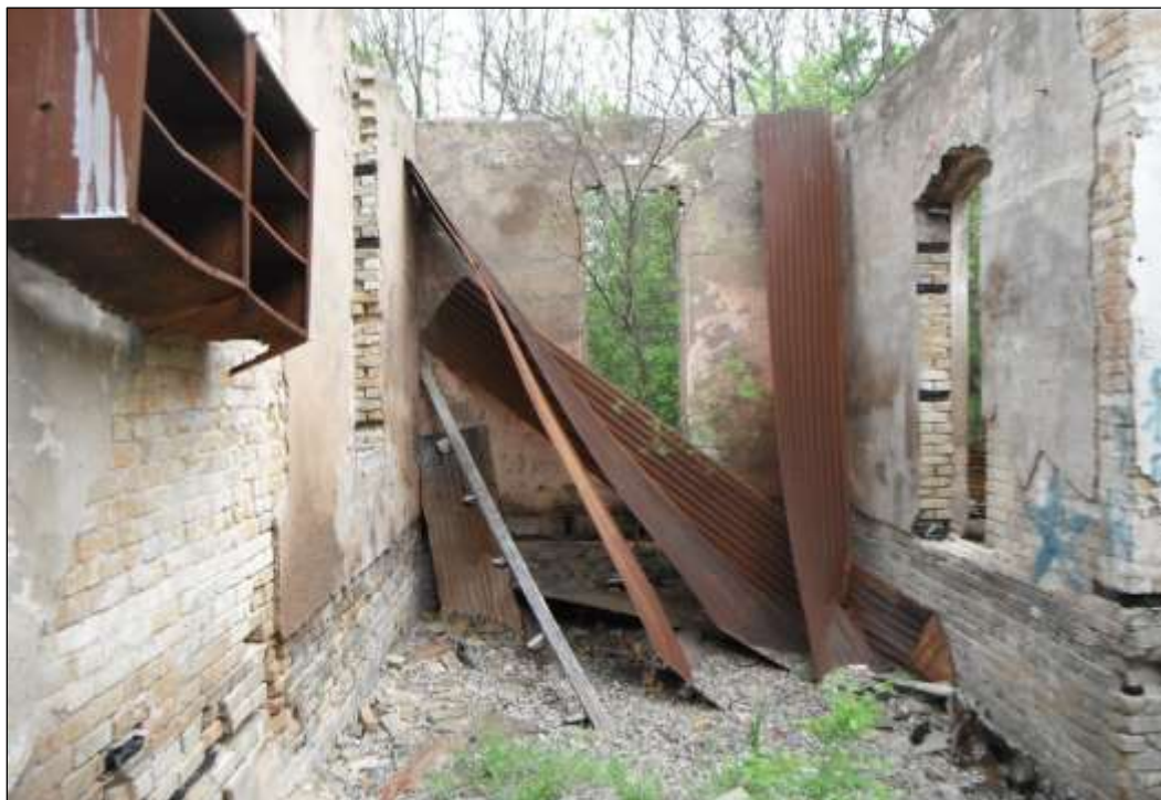
Figure 6-61. Structure W6-A (41HY541)—Northeastern Room Interior (Facing Northeast)
