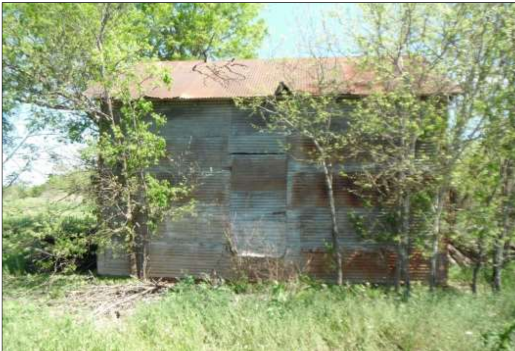
Figure 6-40. Structure W4-B (41HY539)—Side of Barn (Facing Northeast)
