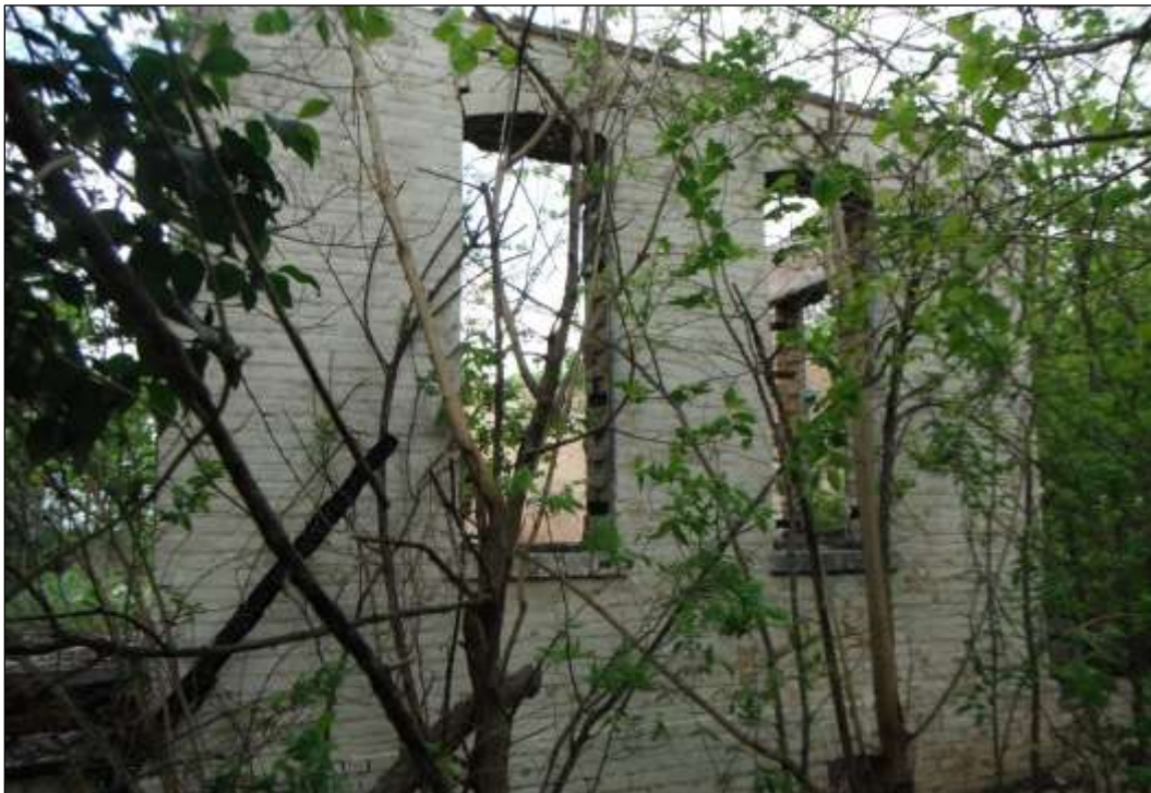
Figure 6-60. Structure W6-A (41HY541)—Southeastern Side of House (Facing West)
