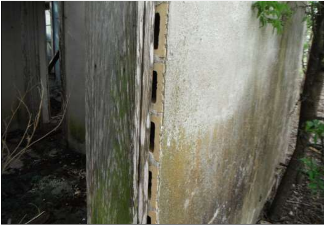
Figure 6-25. Structure W2 (41HY537)—Detail of Clay Tile Construction
