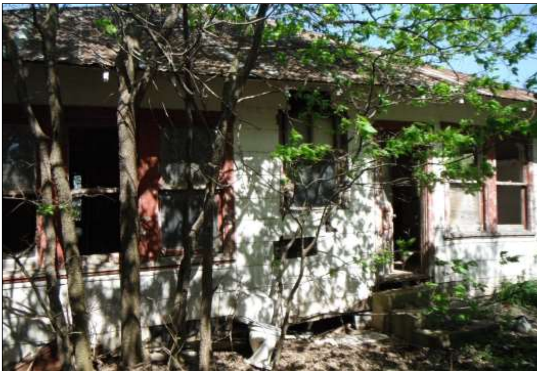
Figure 6-5. Structure W1-A (41HY536)—Rear of House (Facing Northwest)
