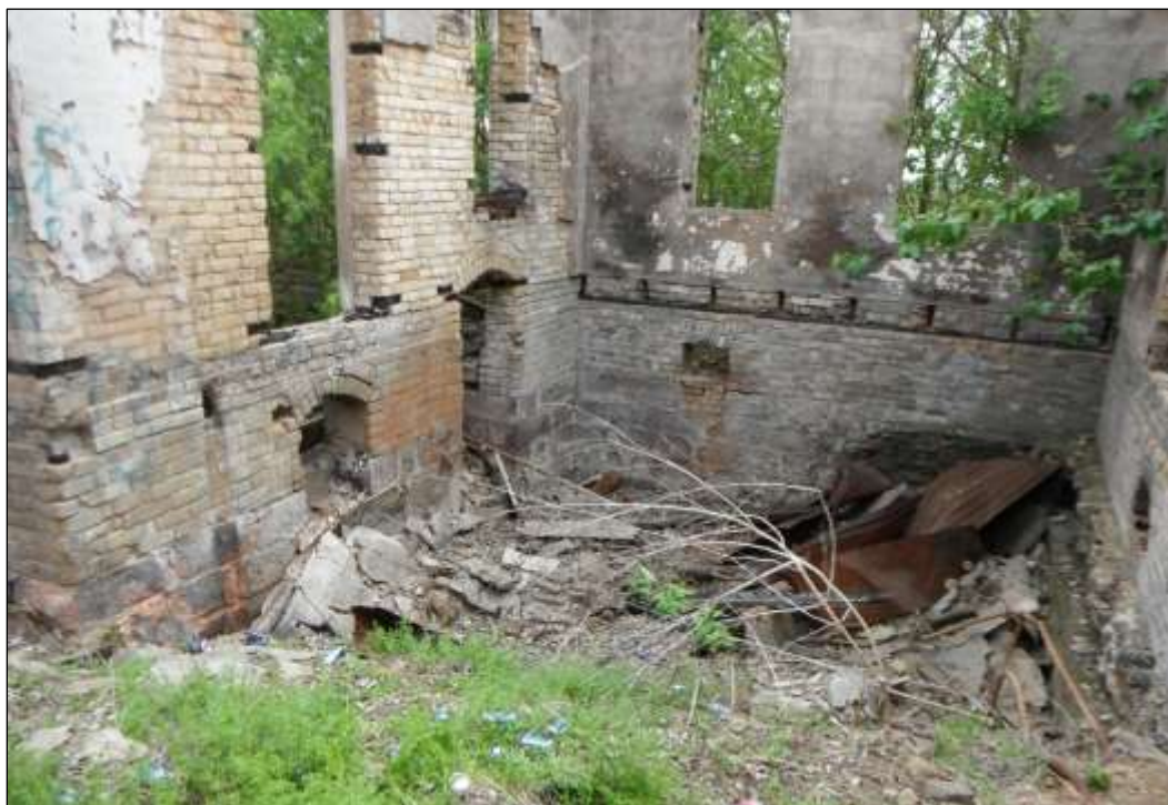
Figure 6-62. Structure W6-A (41HY541)—Southeastern Room and Basement Interior (Facing Southeast)
