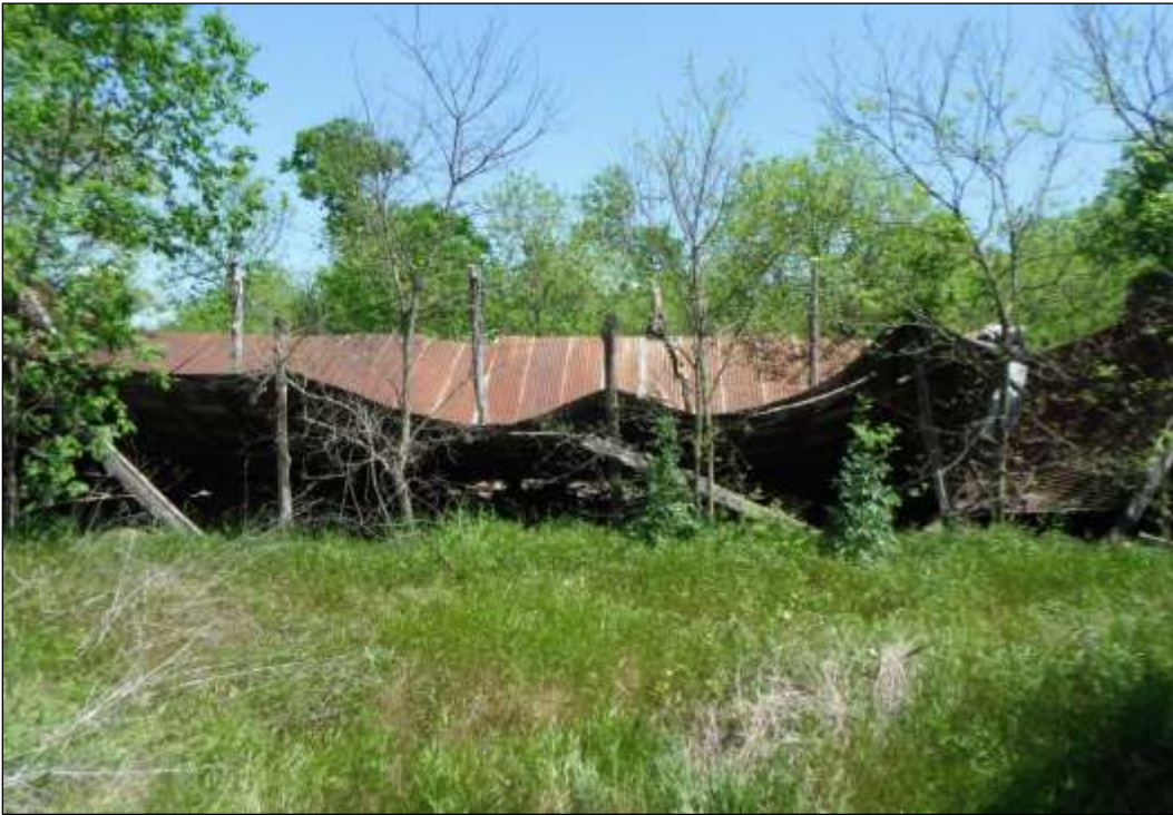
Figure 6-42. Structure W4-C (41HY539)—Southwestern Side of Barn (Facing Northeast)
