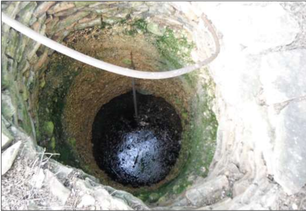
Figure 6-31. Structure W3 (41HY538)—Interior of Well
