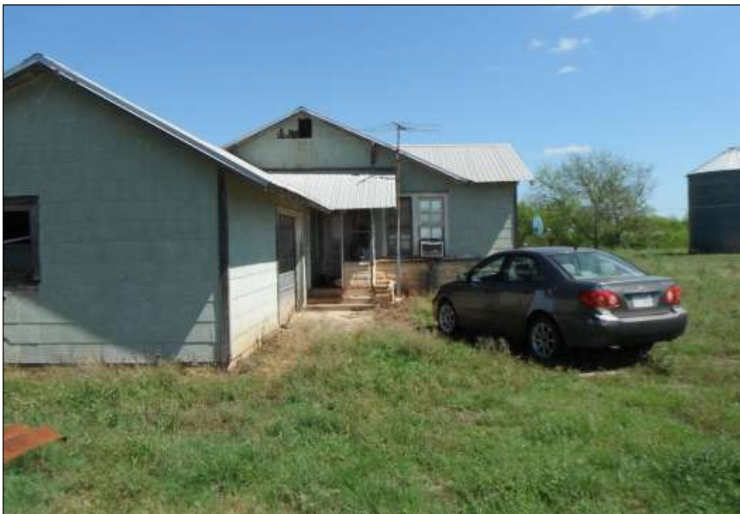
Figure 6-39. Structure W4-A (41HY539)—Back of House (Facing Northeast)
