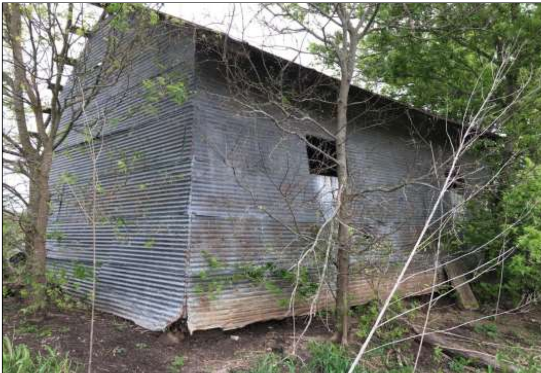
Figure 6-71. Structure W7 (41HY542)—Southwestern Corner of Barn (Facing Northeast)
