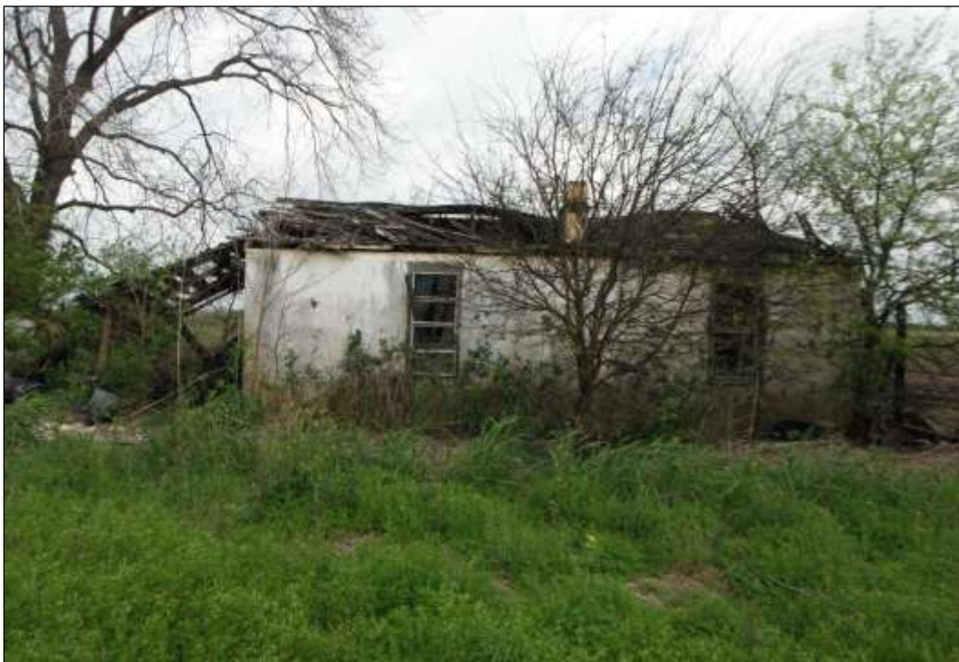
Figure 6-22. Structure W2 (41HY537)—Southeastern Side of House (Facing Northwest)
