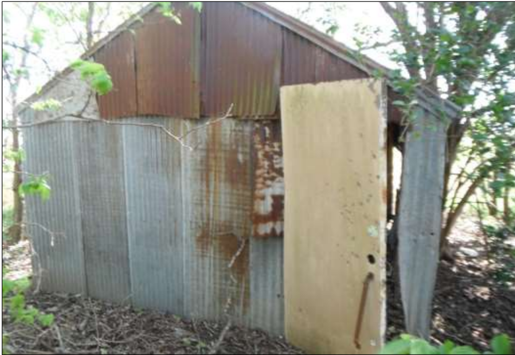
Figure 6-14. Structure W1-E (41HY536)—Side of Eastern Barn (Facing Southeast)
