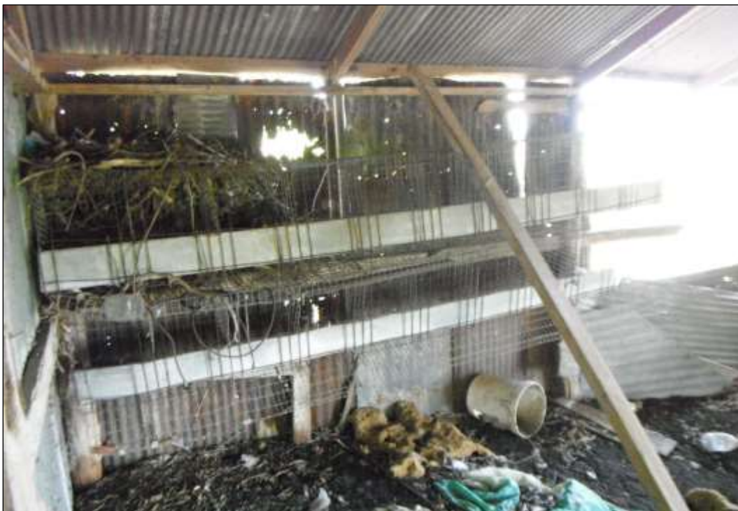
Figure 6-15. Structure W1-E (41HY536)—Interior of Eastern Barn (Facing Northeast)
