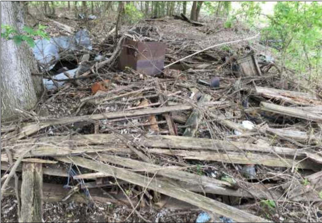
Figure 6-73. Collapsed Structure on Site 41HY542 (Facing Southwest)
