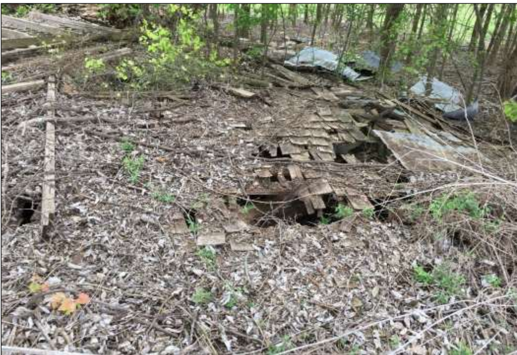
Figure 6-74. Collapsed Roofing of Structure on Site 41HY542 (Facing Southeast)
