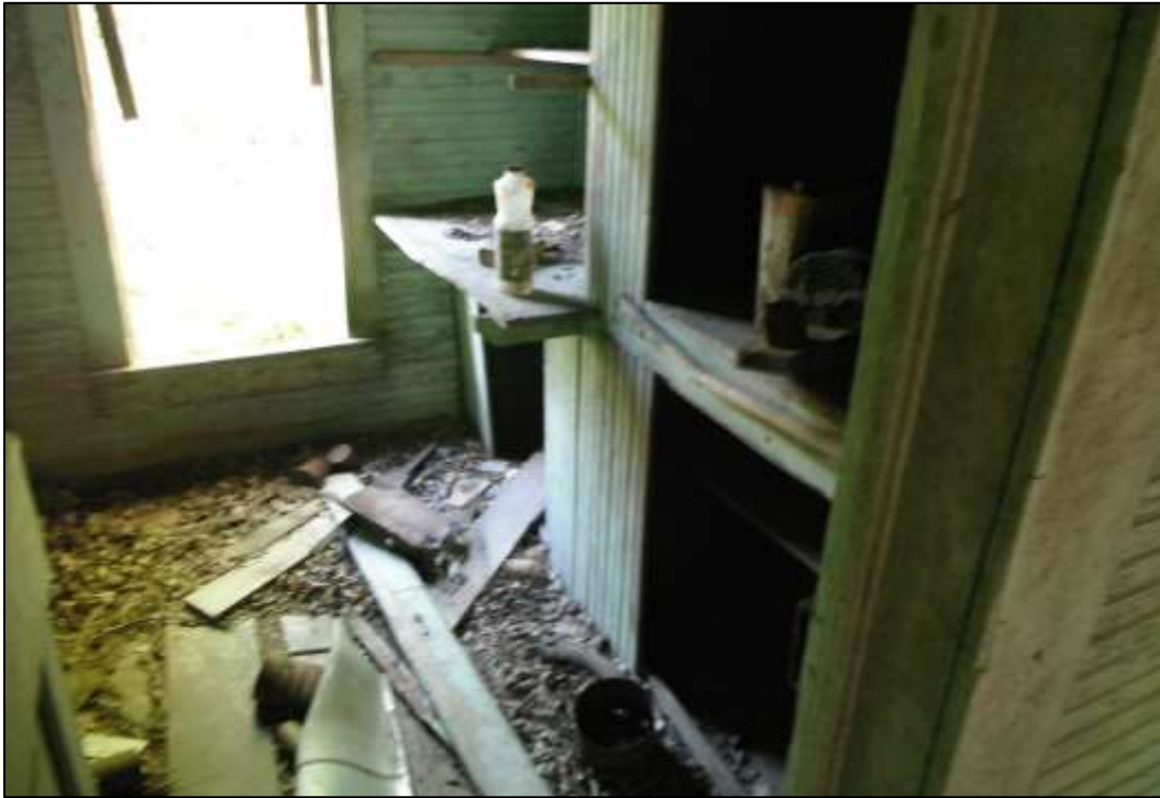
Figure 6-21. Resource 1A—View of Kitchen Pantry (Facing South)
