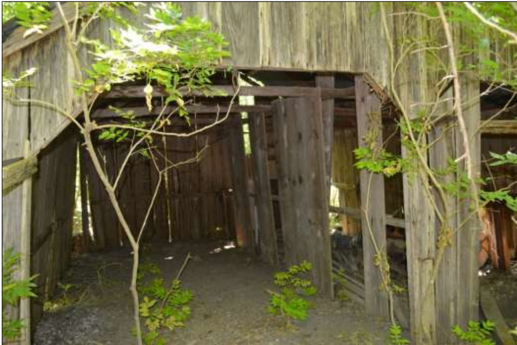
Figure 6-77. Resource 4—Interior of Garage (Facing Northeast)
