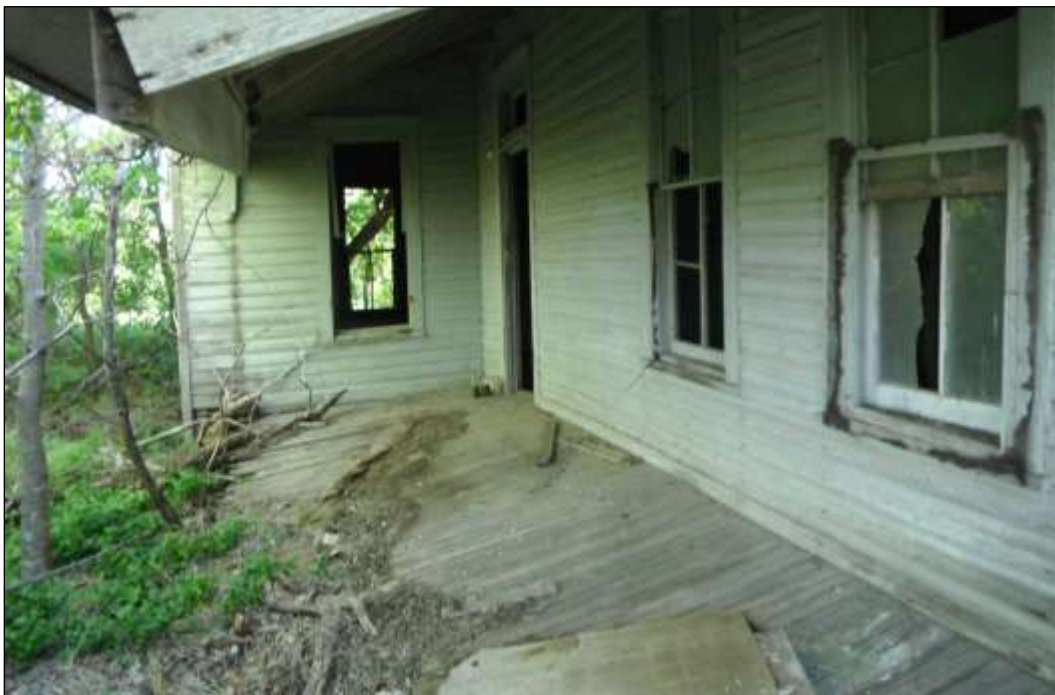
Figure 6-9: Resource 1A—Partial-Width Porch on Western Façade of House (Facing North)
