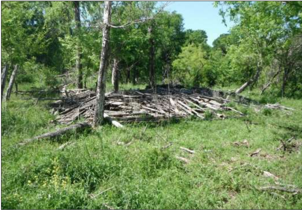
Figure 6-54. Overview of Collapsed Barn on Site 41TV2453 (Facing Southwest)
