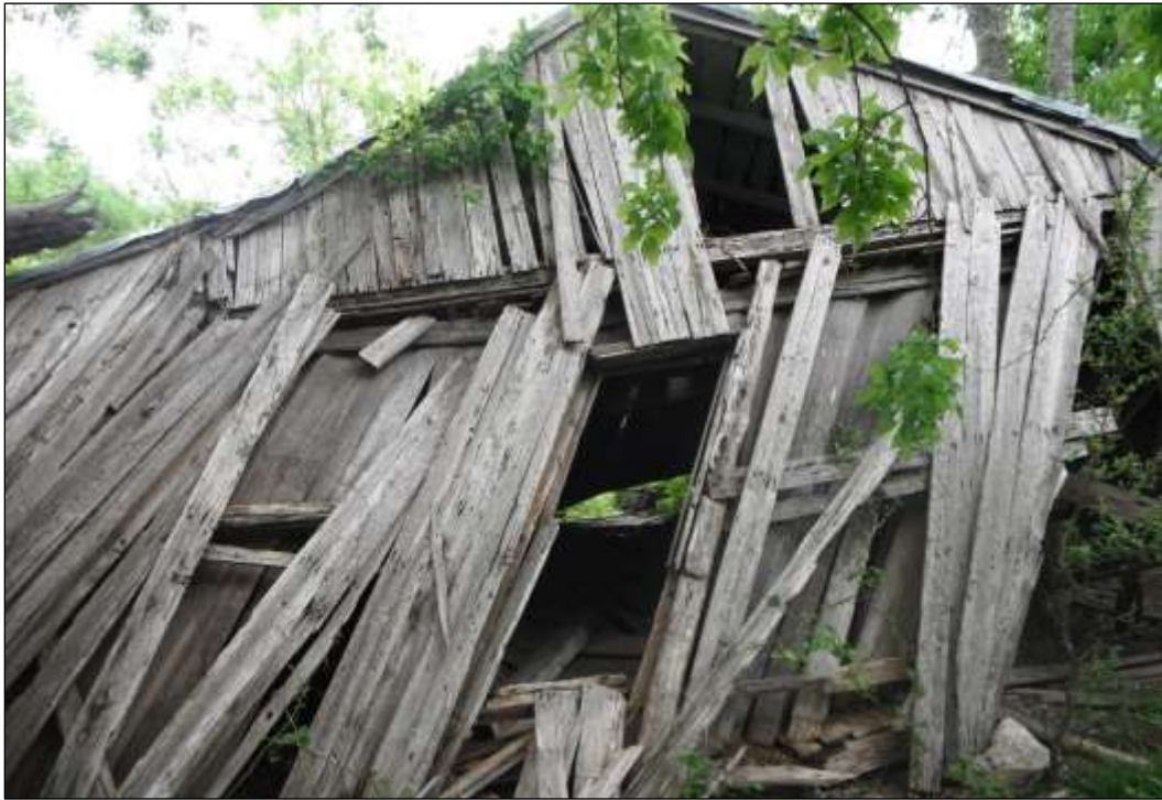
Figure 6-59. Resource 3A—View of the Western Façade of the House (Facing East)
