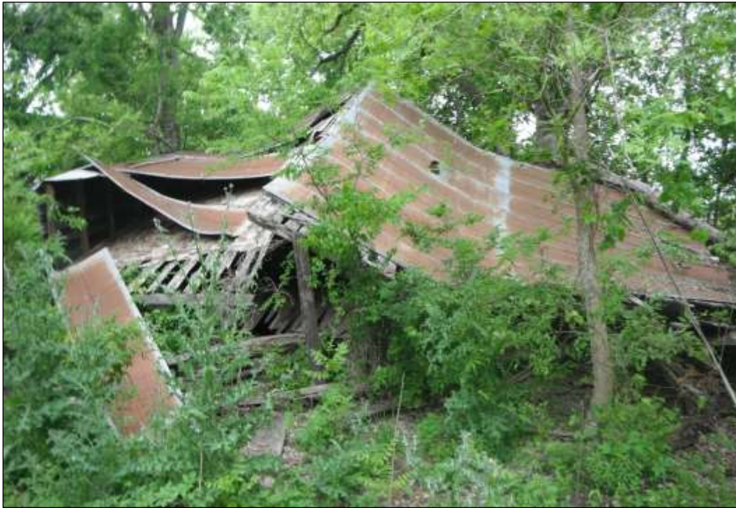
Figure 6-60. Resource 3A—View of the House (Facing West)
