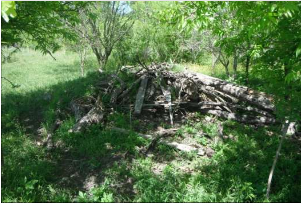
Figure 6-37. View of Debris Pile (Collapsed Former Outbuilding) on Site 41TV2518 (Facing Southwest)
