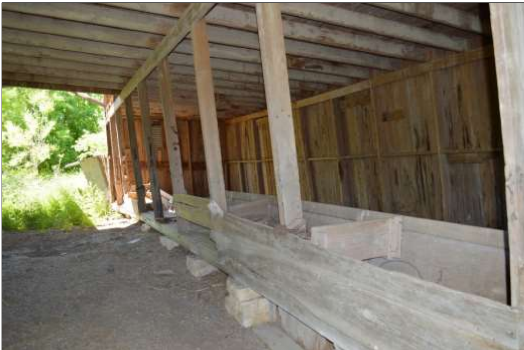
Figure 6-31. Resource 1C—Open Stalls and Feeding Trough along Western Side of Barn Interior (Facing Southwest)
