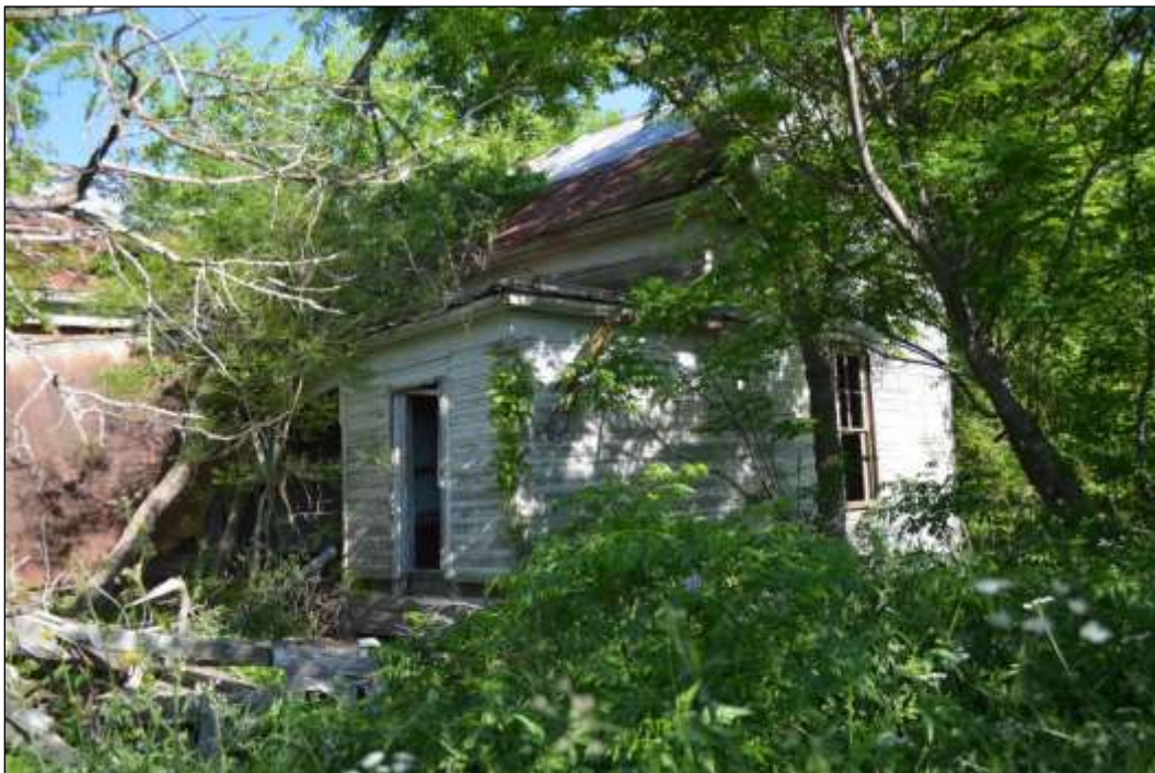
Figure 6-11. Resource 1A—Kitchen Pantry Bump-out at Southeastern Corner of House (Facing Northwest)
