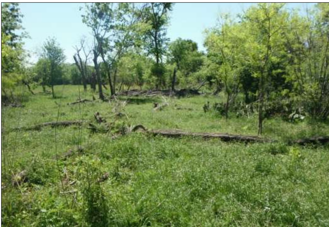
Figure 6-42. View of Collapsed Barn in Clearing on Site 41TV2453 (Facing Southeast)
