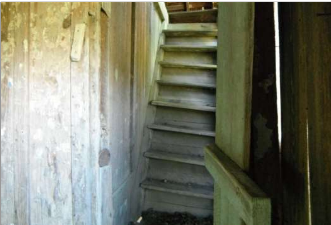
Figure 6-50. Resource 2—View of Interior Enclosed Stairs Leading to Sleeping Loft (Facing South)
