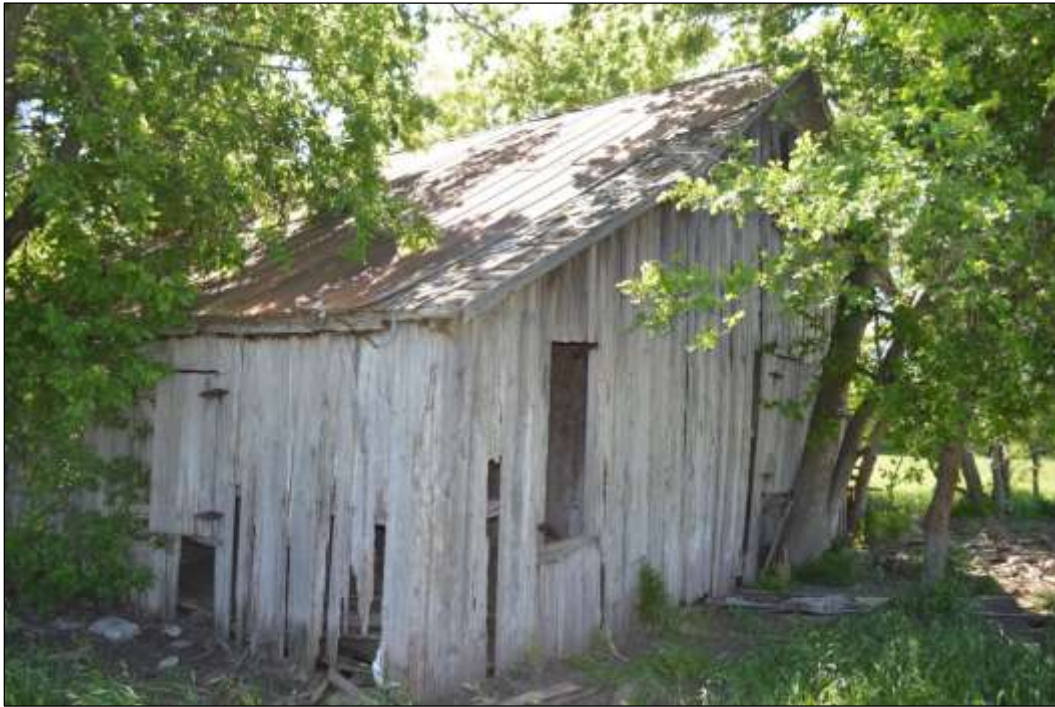
Figure 6-43. Resource 2—View of Western Façade of House (Facing Southeast)
