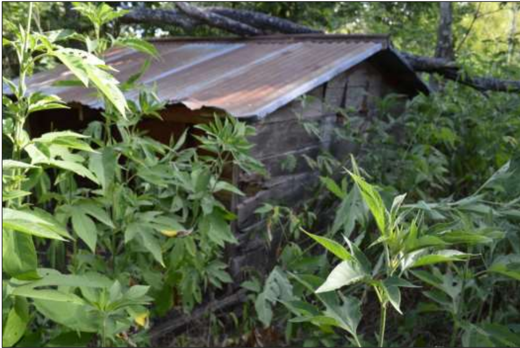
Figure 6-34. Resource 1D—View of Livestock Feeder (Facing Northwest)
