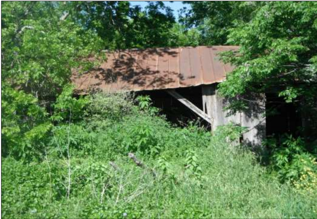
Figure 6-24. Resource 1B—View of Western Façade of Horse Barn (Facing East)
