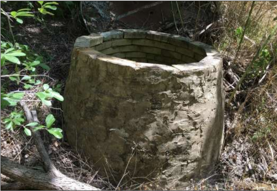
Figure 6-71. View of Stacked Limestone Well on Site 41TV2521 (Facing Southwest)
