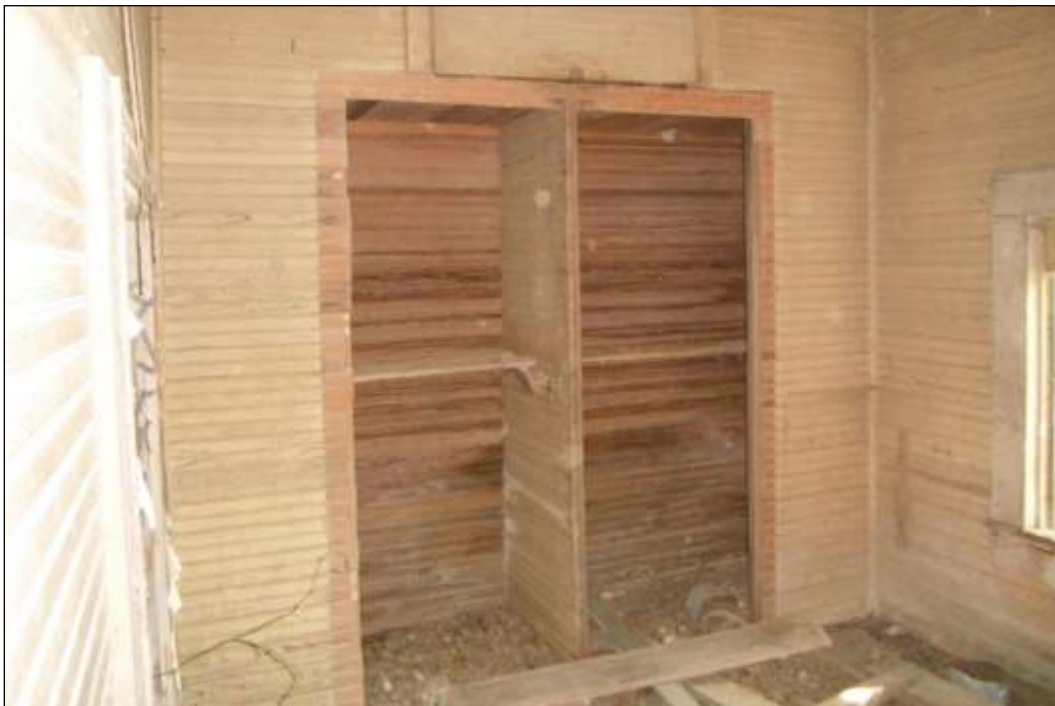
Figure 6-18. Resource 1A—View of Child's Bedroom (Facing Northeast)
