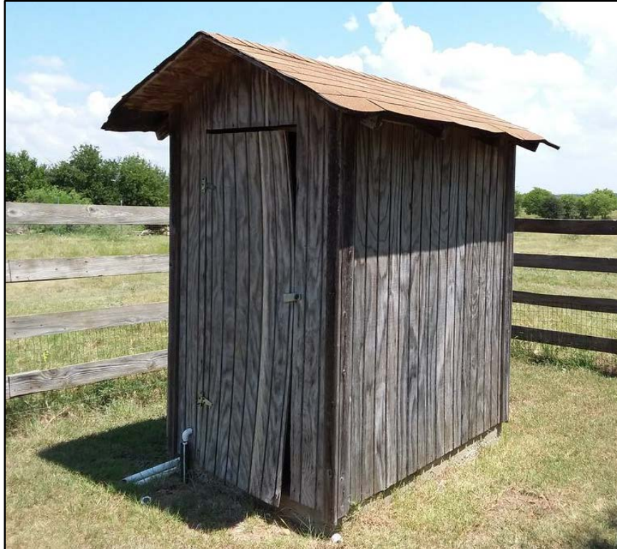
Figure 14b. Wood plank shed with asphalt shingle roof, view northeast.
