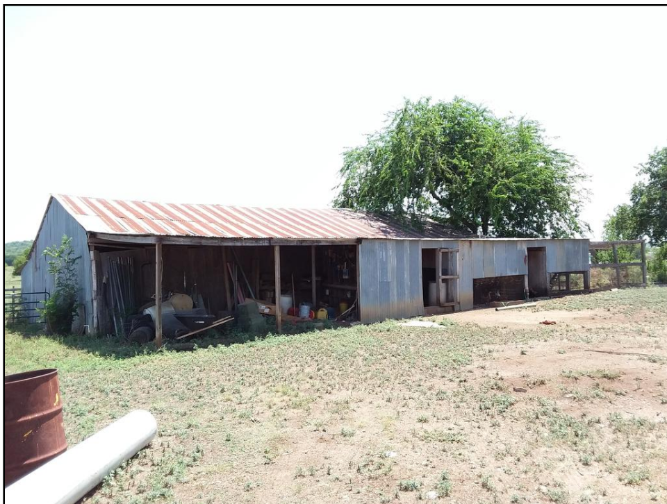
Figure 13. Wood frame barn within the project area, view southwest.
