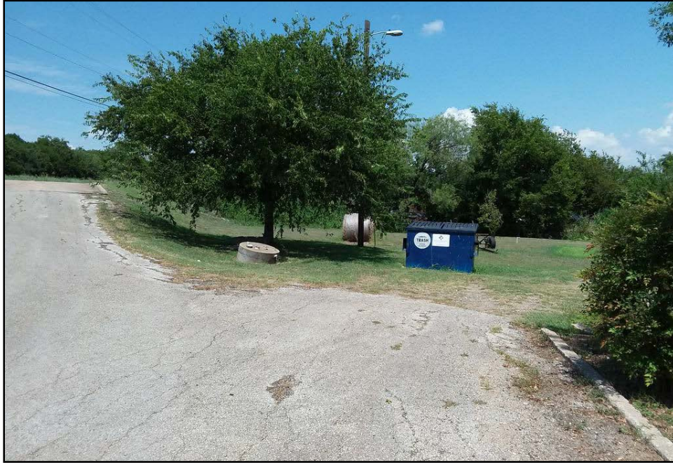
Figure 6. Overview along McKinney Falls Parkway of buried and aboveground utilities, view north.
