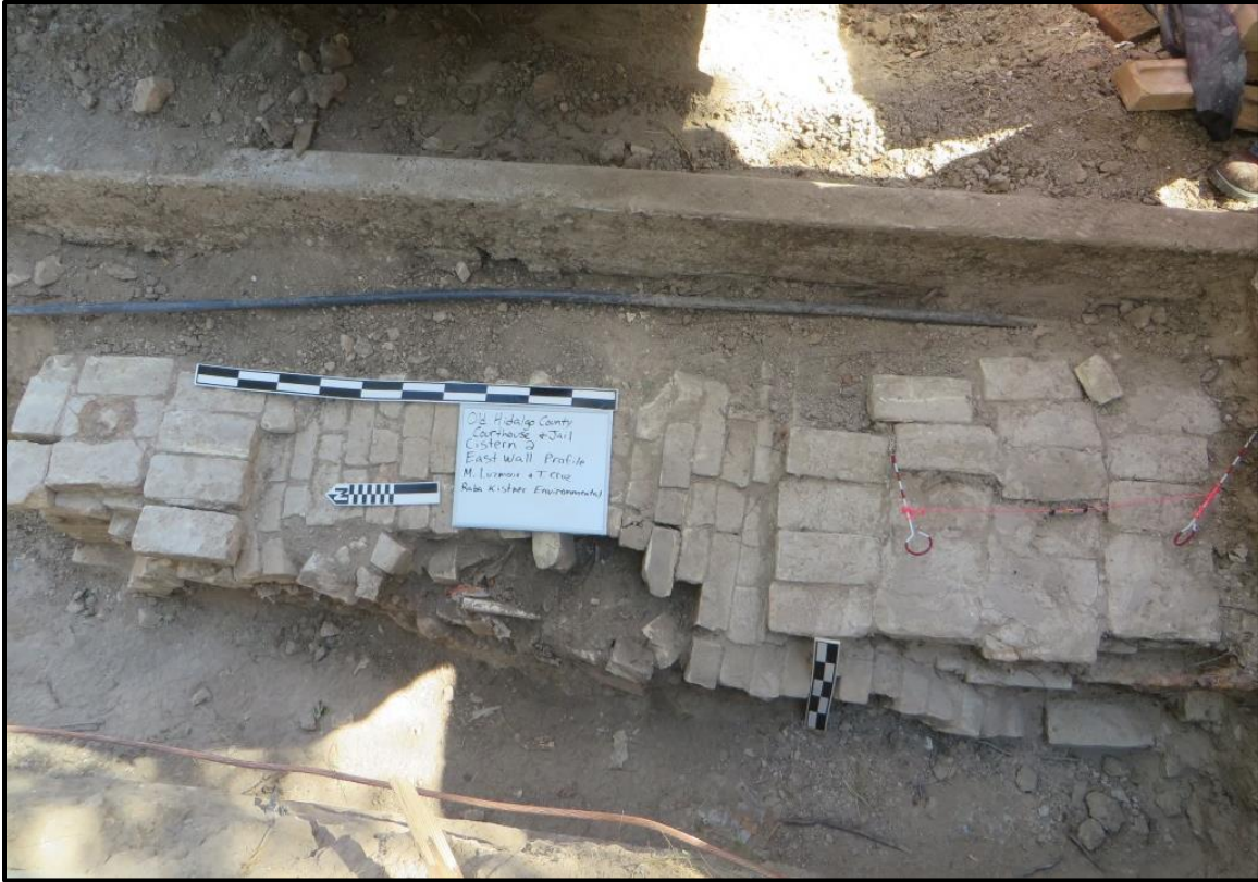
Figure 4-6. Plan view of Cistern 2 after re-exposure. Note metal pipe running along the top.
