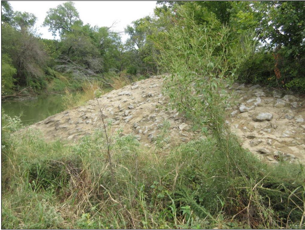
Figure 5: Bank stabilization along the Elm Fork at the South launch; facing south.
