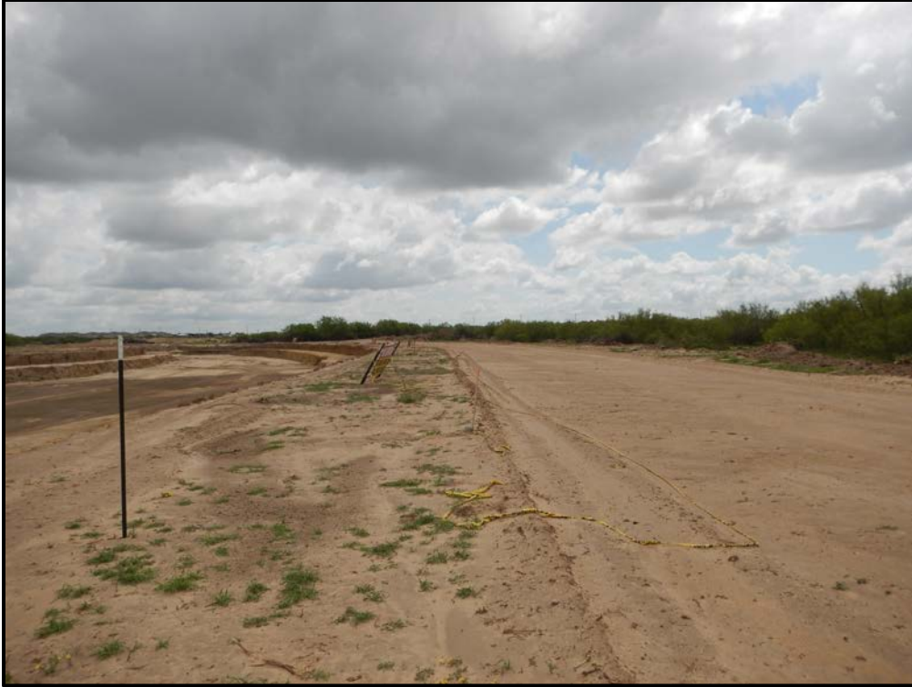
Figure 6. Cleared/scraped portion of proposed APE (see Figure 9-2 for location where photograph was taken).
