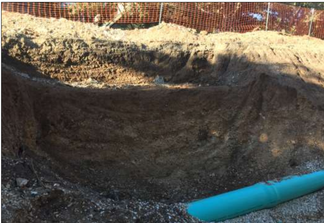
Figure 20. Profile 2 of Alluvial Gravels at Active Construction Site (Facing South)
