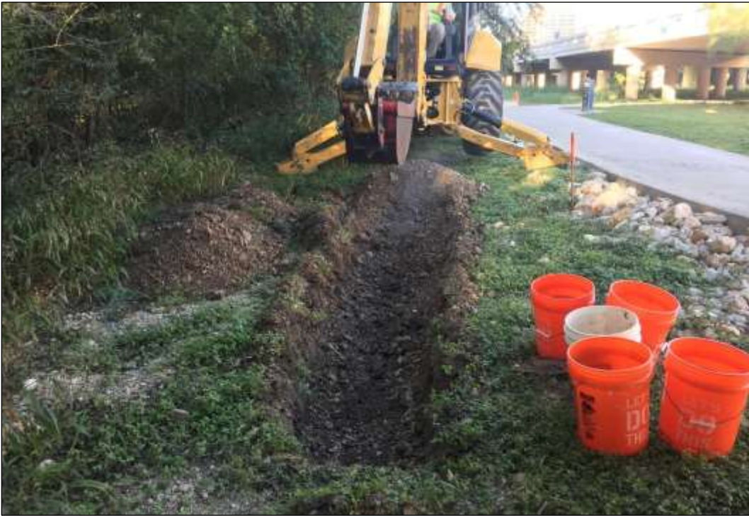
Figure B-1. Photographic Overview of BHT-1 (Facing West)
