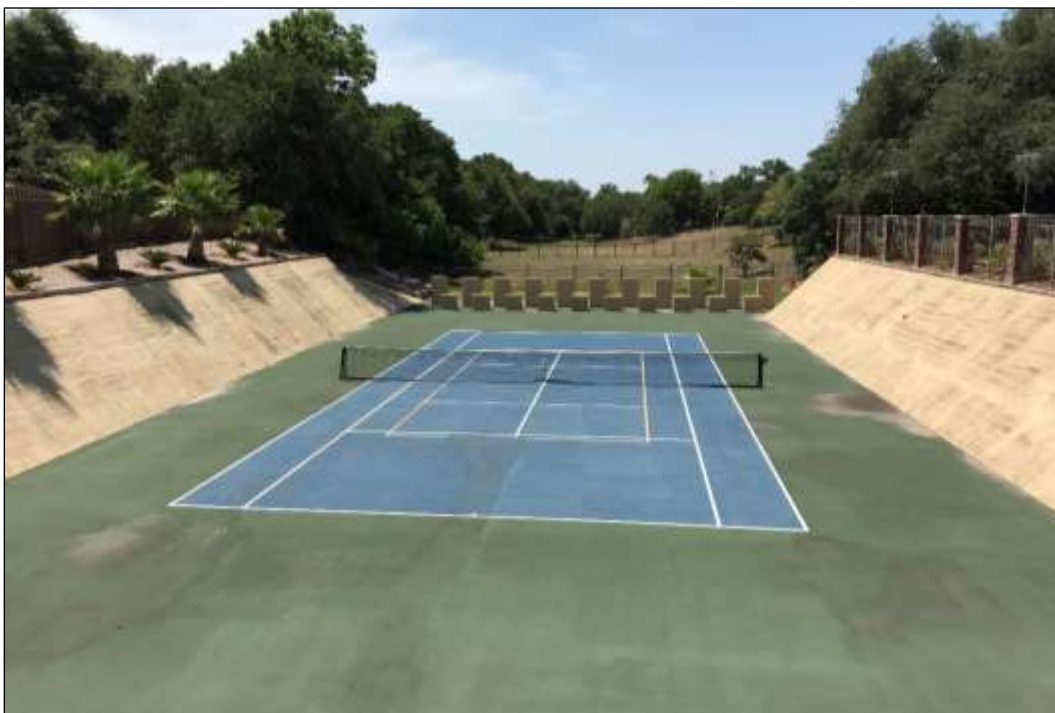
Figure 13. Storm Water Detention Basin within Northern Portion of Project Area (Tennis Court Installed by Local Landowner) (Facing South)
