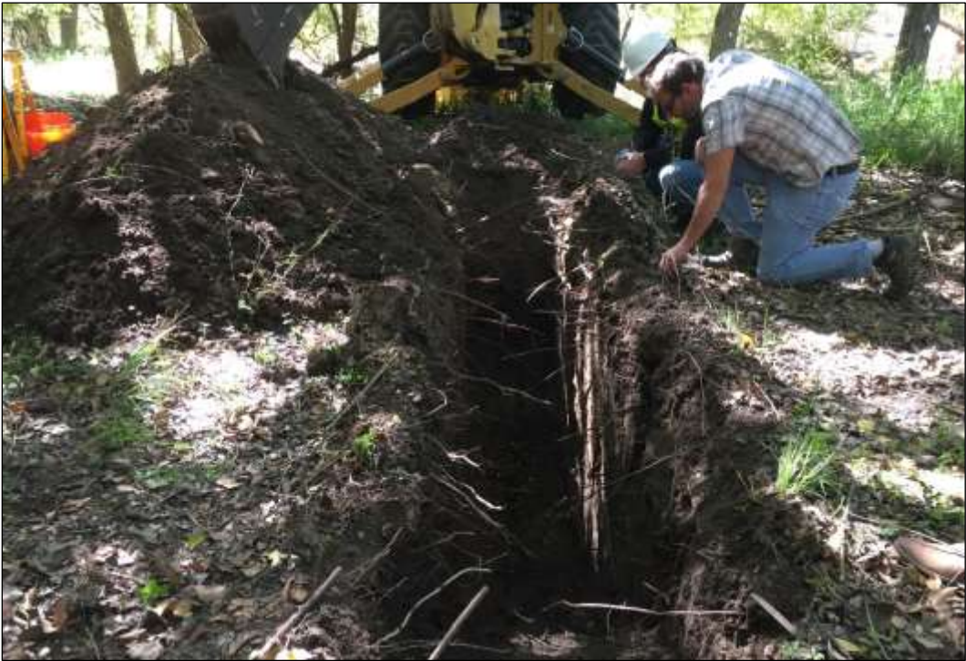
Figure B-5. Photographic Overview of BHT-3 (Facing West)
