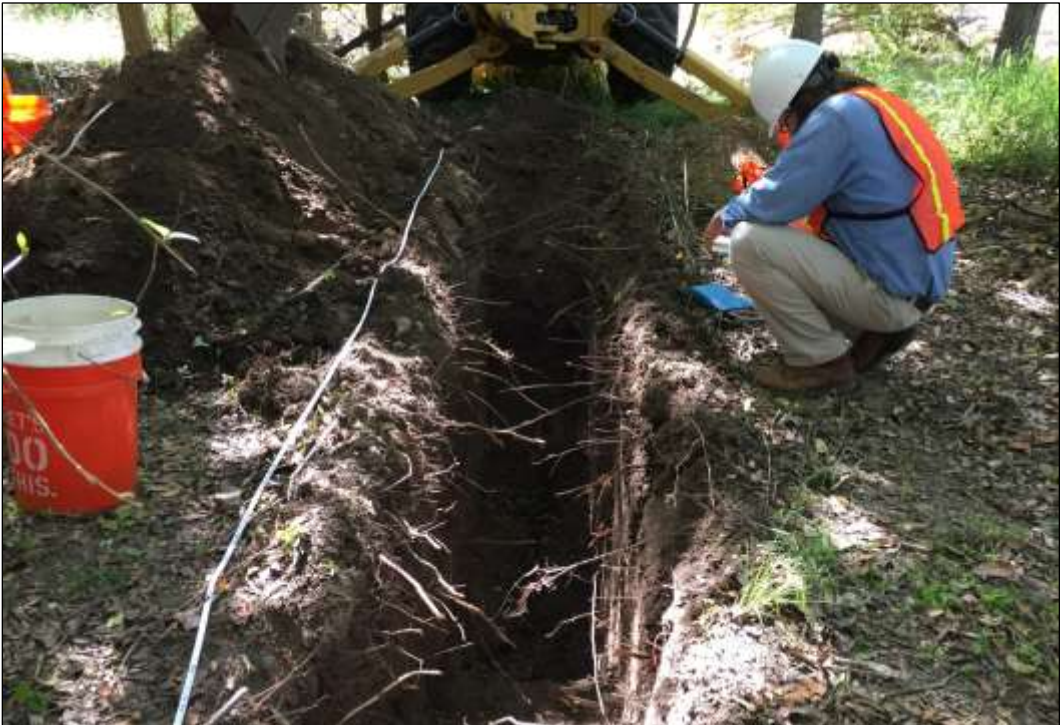
Figure B-6. Close-up View of BHT-3 (Facing West)
