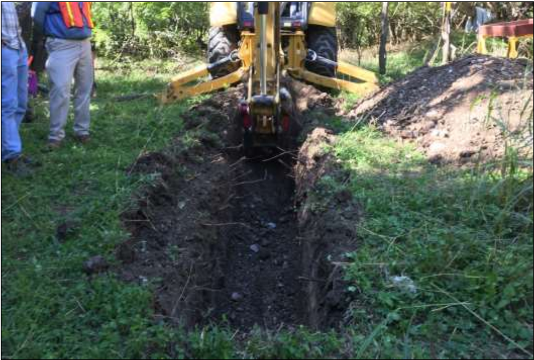
Figure B-3. Photographic Overview of BHT-2 (Facing West)
