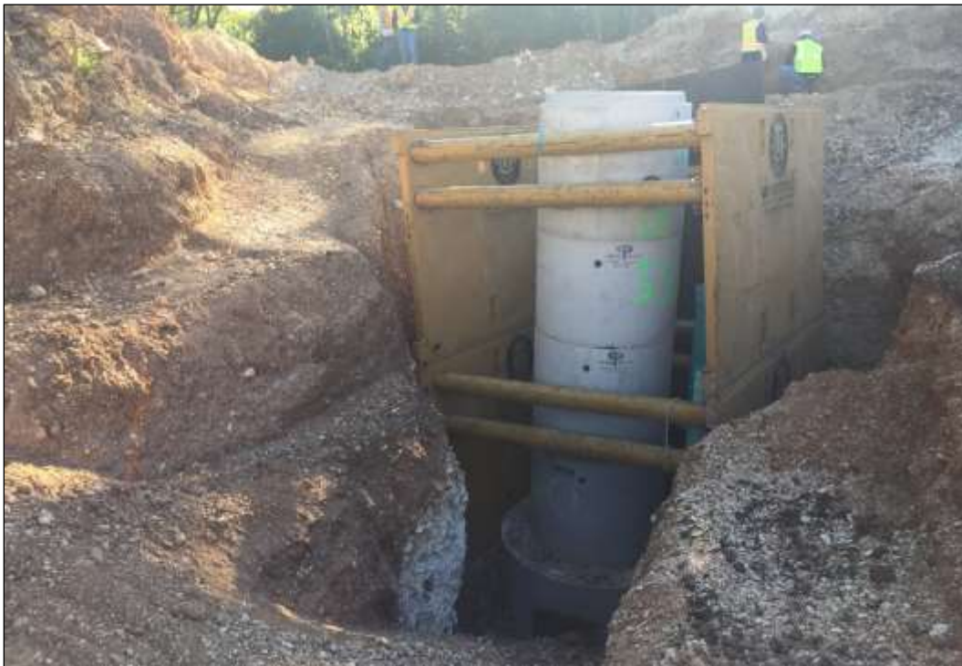
Figure 18. Sewer Manhole under Construction along Ira Lee Road (Facing West)
