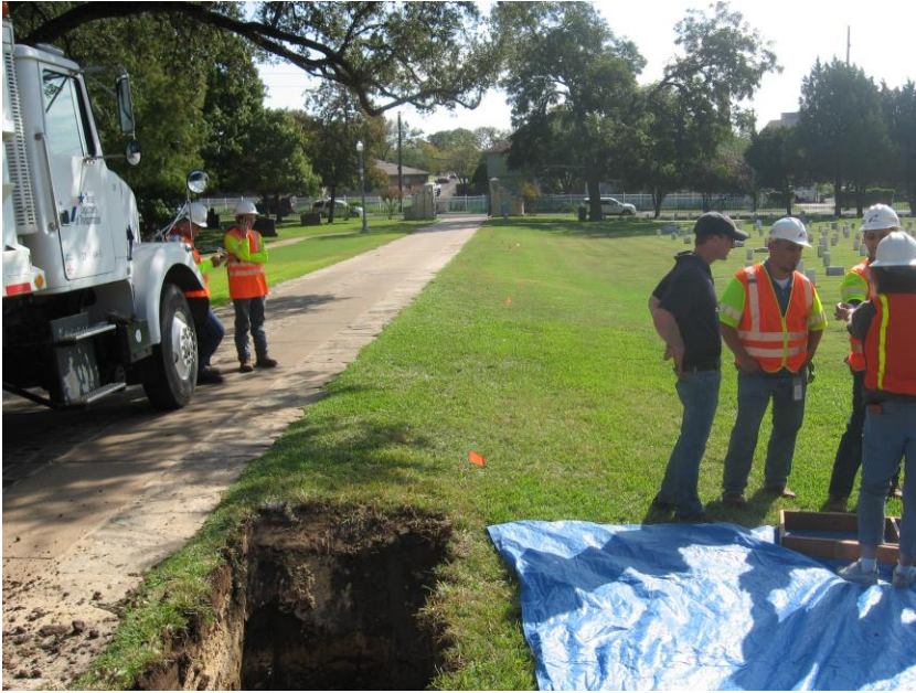
Photo #3: Facing east toward Gradall Trench (GT) #1.
