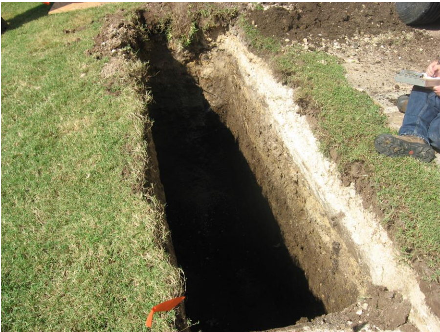
Photo #5: Facing west toward Gradall Trench GT #2. Note the fill levels in the right hand side of the frame.
