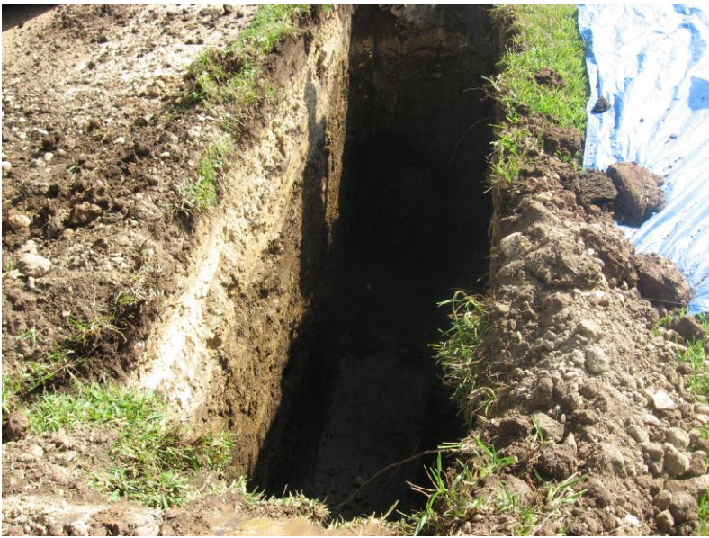
Photo #3: Facing east toward Gradall Trench (GT) #1.
