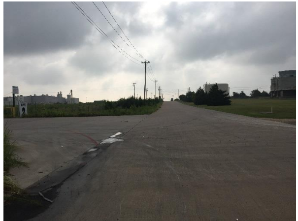
Photograph 10 – Looking East – Active Road
