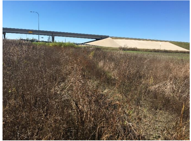
Photograph 2 – Looking West – General Overview
