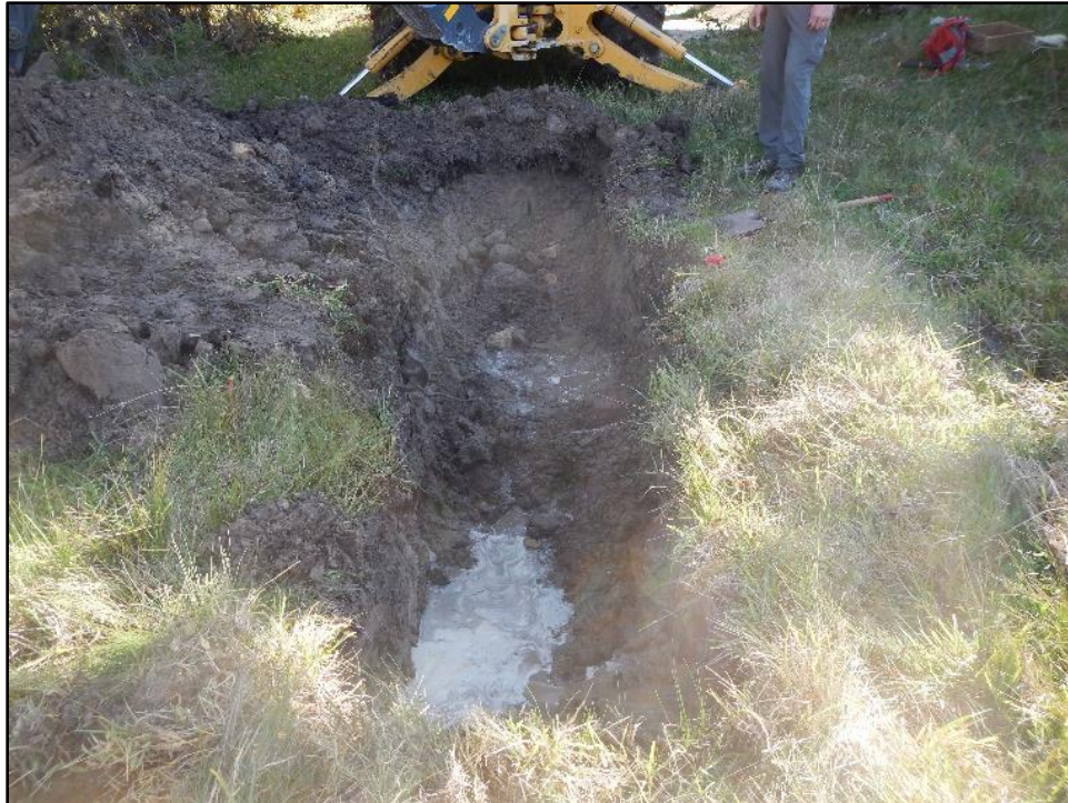
Figure 8. Backhoe Trench 4 showing shallow water table in East Mill Creek floodplain.
