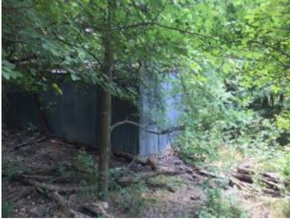
Photograph 37 - 41TV2542 Feature 2 Looking Northeast
