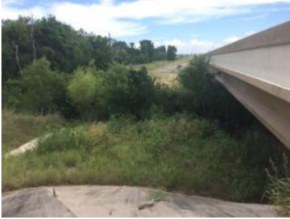
Photograph 79 - General Photo Looking North
