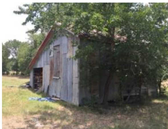
Photograph 28 - 41TV2542 Feature 1 Looking Southeast
