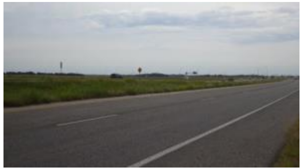
Photograph 10 - General Photo Looking Southwest
