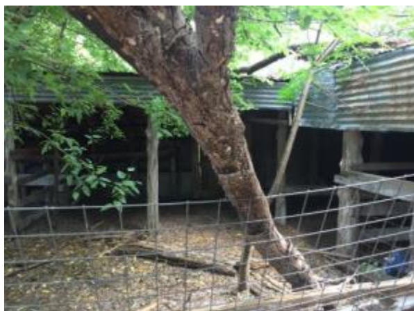
Photograph 47 - 41TV2542 Feature 3 Looking South
