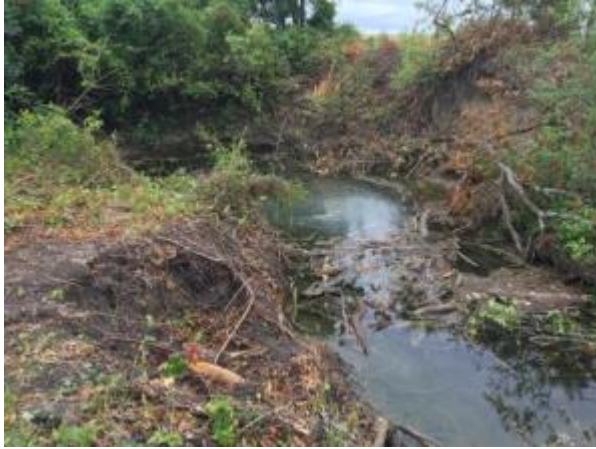
Photograph 19 - General Photo Looking Northeast
