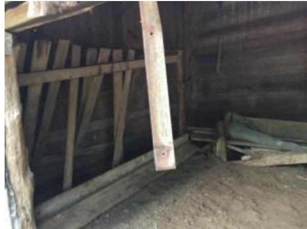
Photograph 52 - 41TV2542 Feature 3 Looking South
