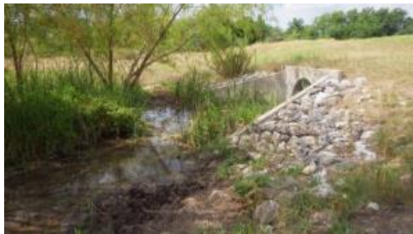
Photograph 6 - General Photo Looking Northwest
