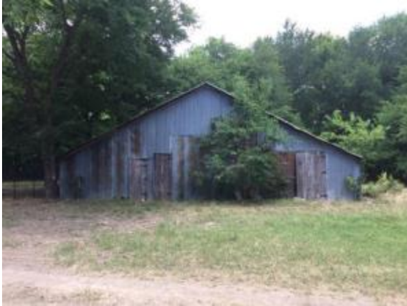
Photograph 33 - 41TV2542 Feature 2 Looking South
