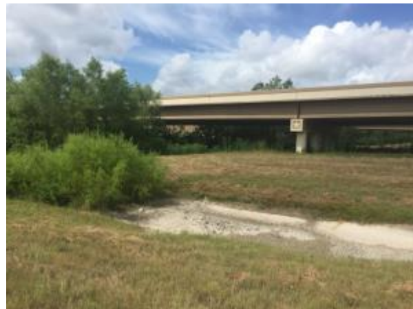
Photograph 78 - General Photo Looking Southwest
