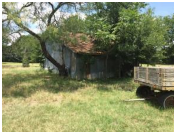
Photograph 30 - 41TV2542 Feature 1 Looking Northeast
