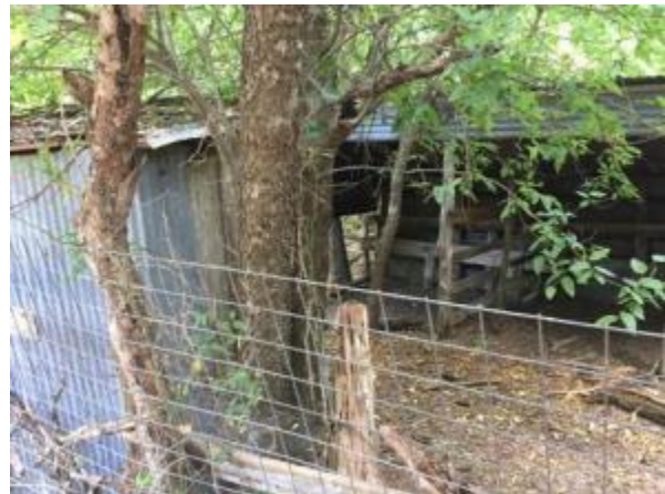
Photograph 54 - 41TV2542 Feature 4 Looking Southeast
