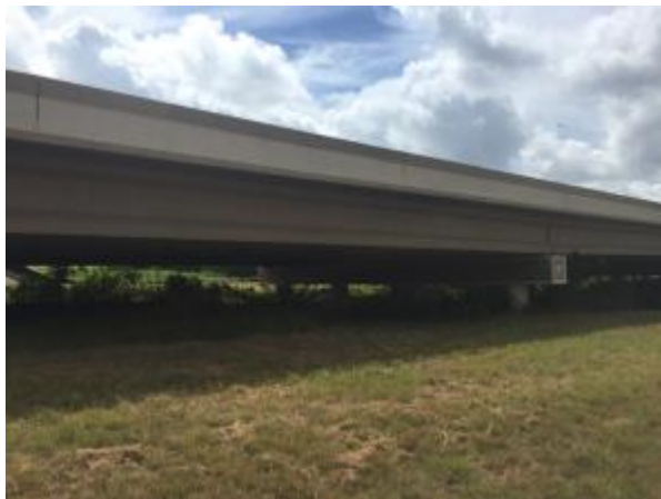
Photograph 77 - General Photo Looking Northwest
