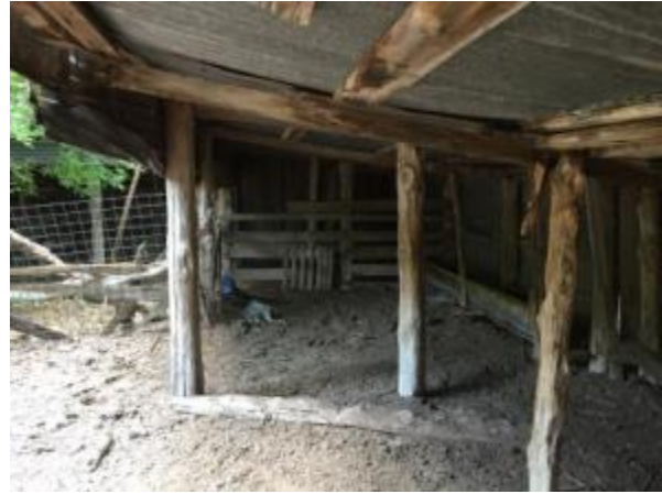
Photograph 50 - 41TV2542 Feature 3 Looking South
