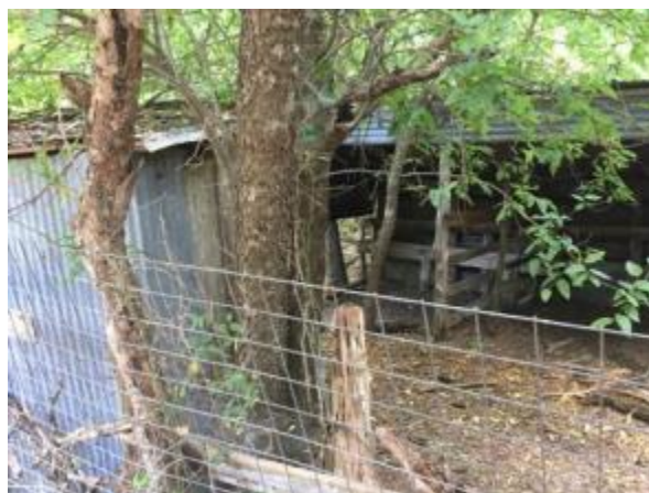
Photograph 48 - 41TV2542 Feature 3 Looking Southeast
