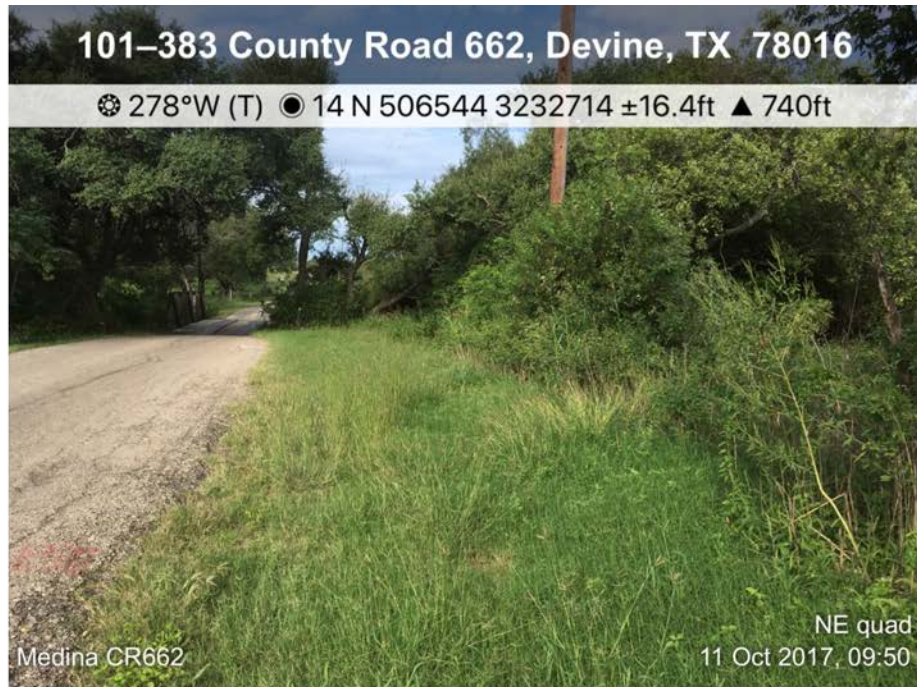
Figure 15. North abutments vegetation at fence line.
