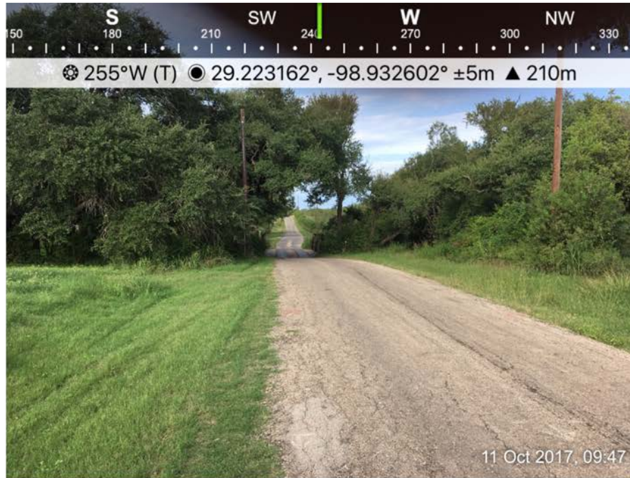
Figure 11. Overview of roadway showing elevated section.
