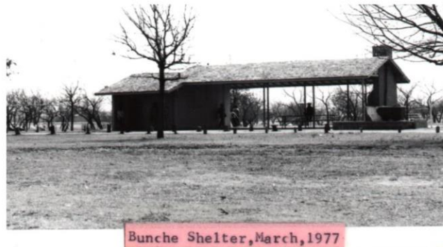
Figure 24: Bunche Park Shelter, March 1977. Since demolished. Courtesy Fort Worth Park and Recreation Department.
