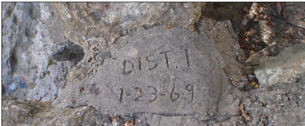
Figure 17. Date inscribed in the mortar on the culvert (41TR306).
