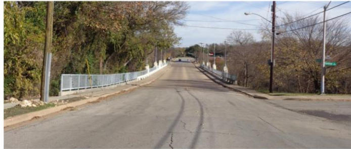
Figure 1: View of the Park Hill Drive Bridge looking east from Sandage Avenue.
