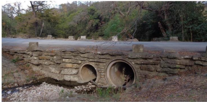
Figure 5: West side of culvert. Looking east/northeast.
