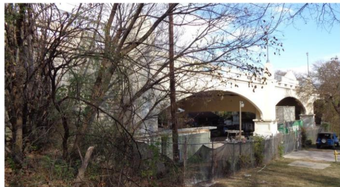
Figure 3: View of south side of bridge from embankment. Looking northeast.
