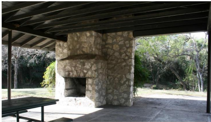
Figure 12: Stone fireplace and exposed roof trusses. Looking northwest.
