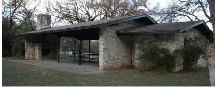
Figure 11: West and south elevations of the Forest Park Shelter. Looking northeast.
