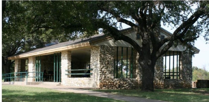
Figure 22: Oakland Lake Park shelter. Designed by Robert P. Woltz, Jr. and constructed by park department employees in 1953.
