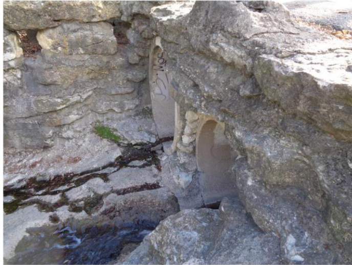
Figure 6: East side of culvert. Looking south.
