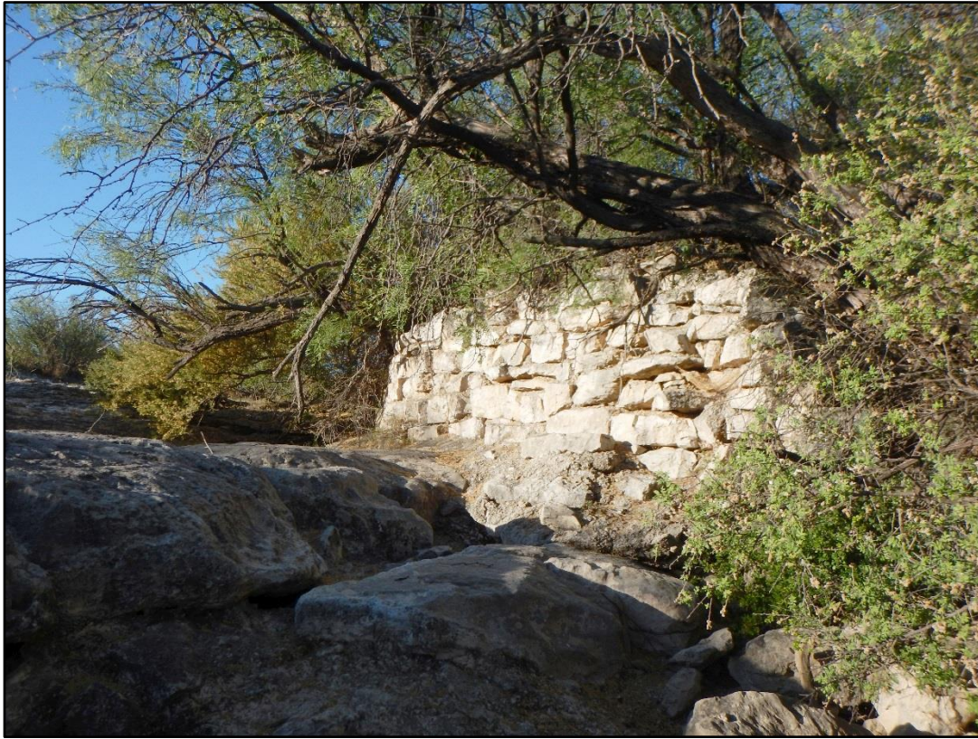
FIGURE 4-12. Site 41PC817 Feature 3 (stone retaining wall and limestone bedrock spillway), facing southeast.
