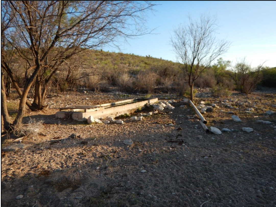
FIGURE 4-11. Site 41PC817 Feature 2 (concrete trough), facing north.
