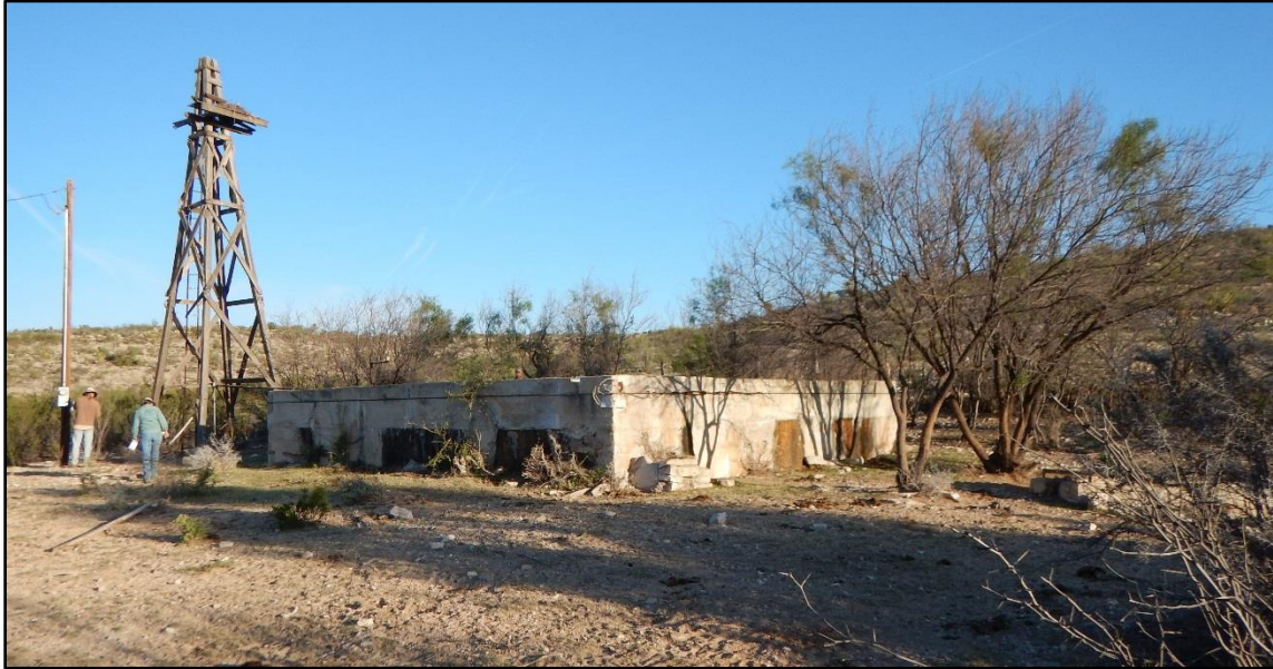
FIGURE 4-9. Site 41PC817 Feature 1 (windmill derrick and concrete tank), facing west.
