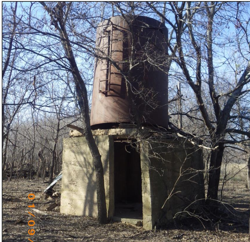
Figure 14. Structure with tank outside the survey corridor. View is to the southwest.
