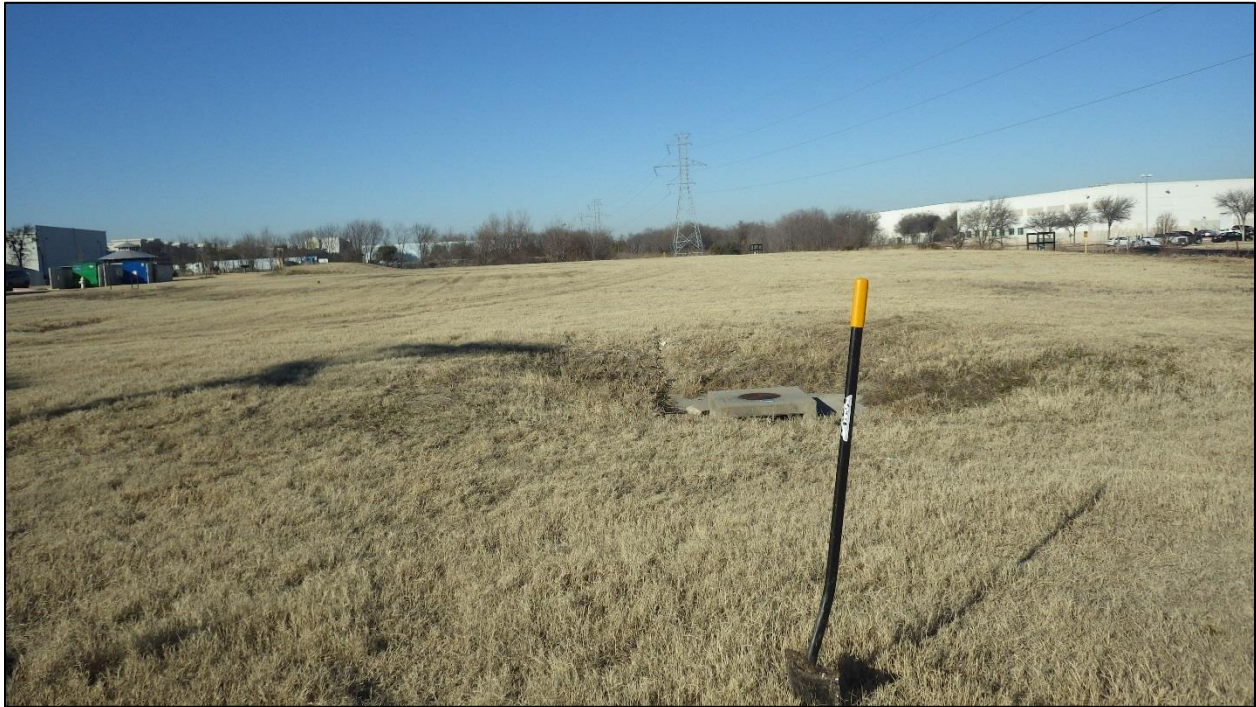
Figure 5. Shortest segment of surveyed pipeline route showing existing utility disturbance, located approximately 20 meters south of Beck Branch. View is facing to the west.
